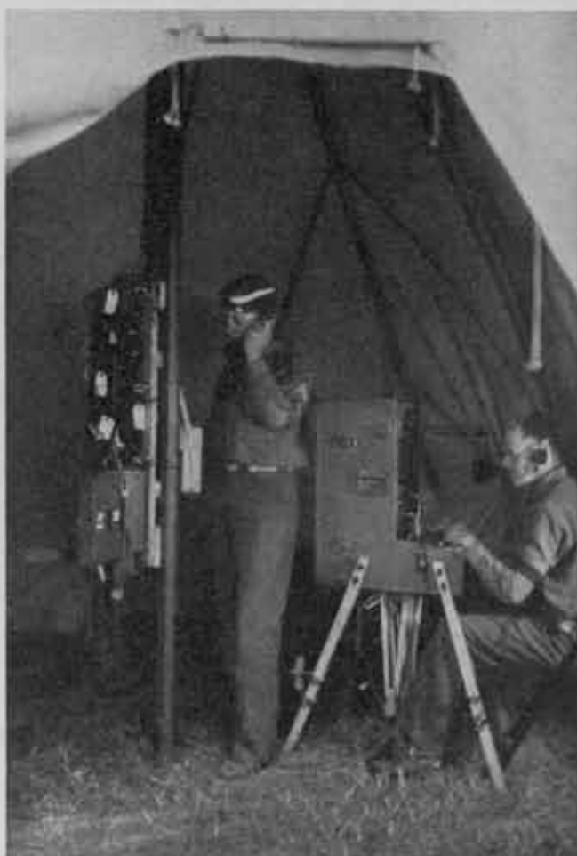
Umpire switchboard at Sterlingville
