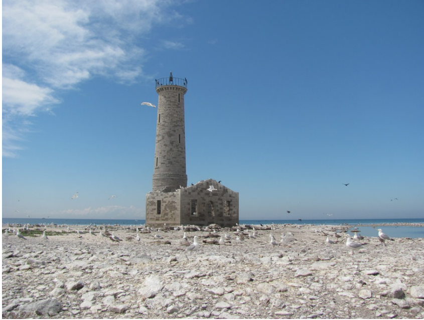
Figure 7: Lighthouse, Mohawk Island National Wildlife Area, 2012
