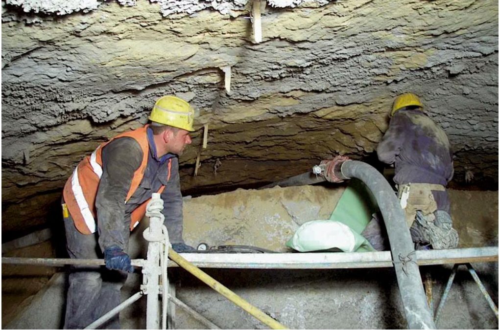
Fig. G.16 Backfill of the precut with pumped mortar
