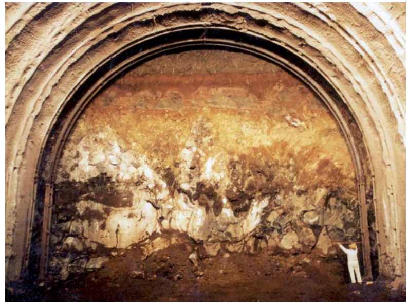
Massimo Tunnel. Passage under the crater of a volcano, overburden: ~ 15 m
