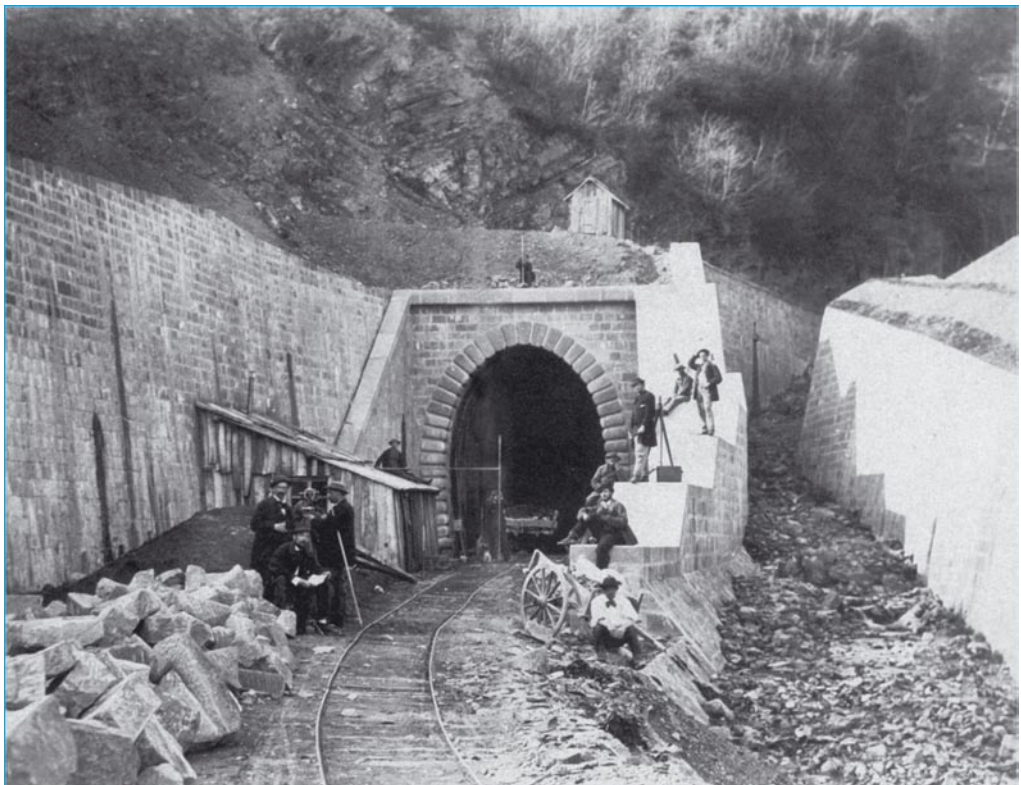
"Porrettana" Line: Construction of the South portal of the Signorino tunnel (1862 ca.)
