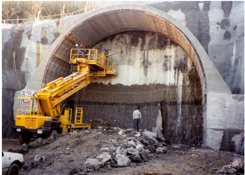
Macchia Piana Tunnel. Work on the north portal (ground: rubble)
