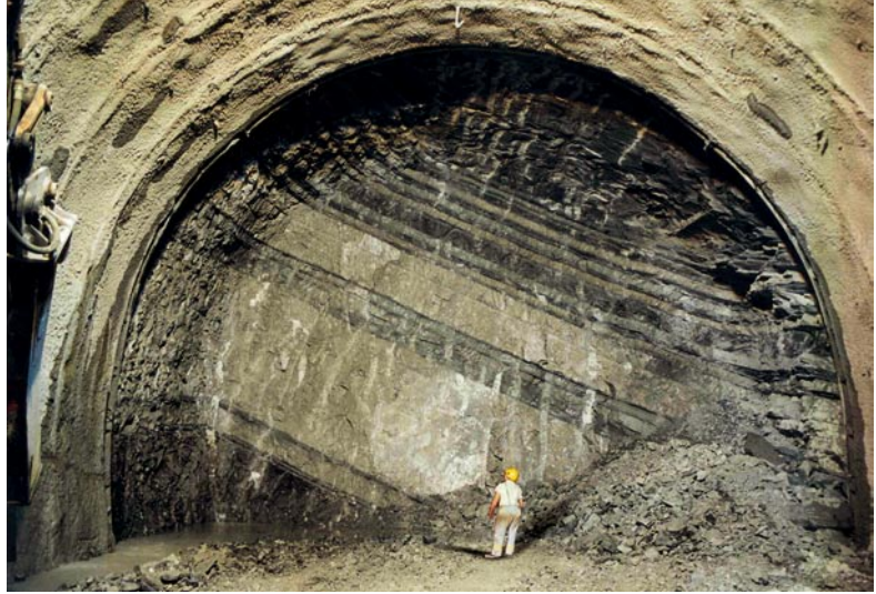
Vaglia Tunnel. View of the face while tunnelling through the Monte Morello formation (overburden: ~ 600 m)
