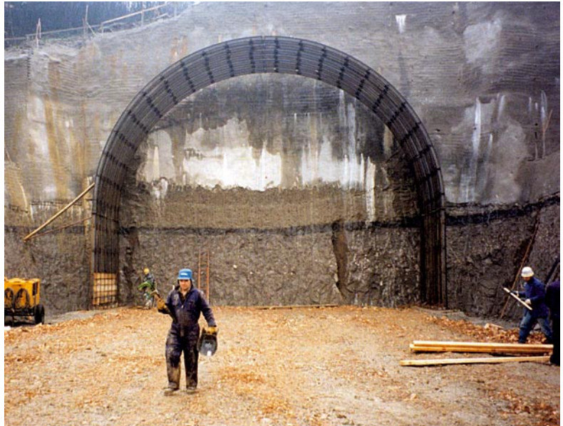
Macchia piana Tunnel. The scaffolding template for the North portal
