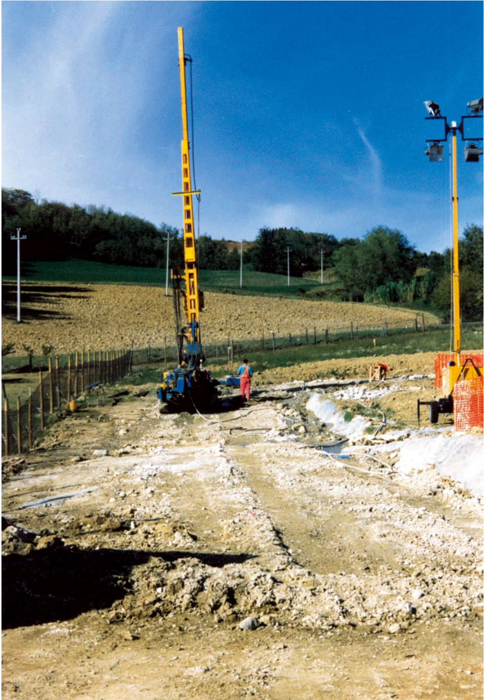
Vertical jet-grouting for a portal shell
