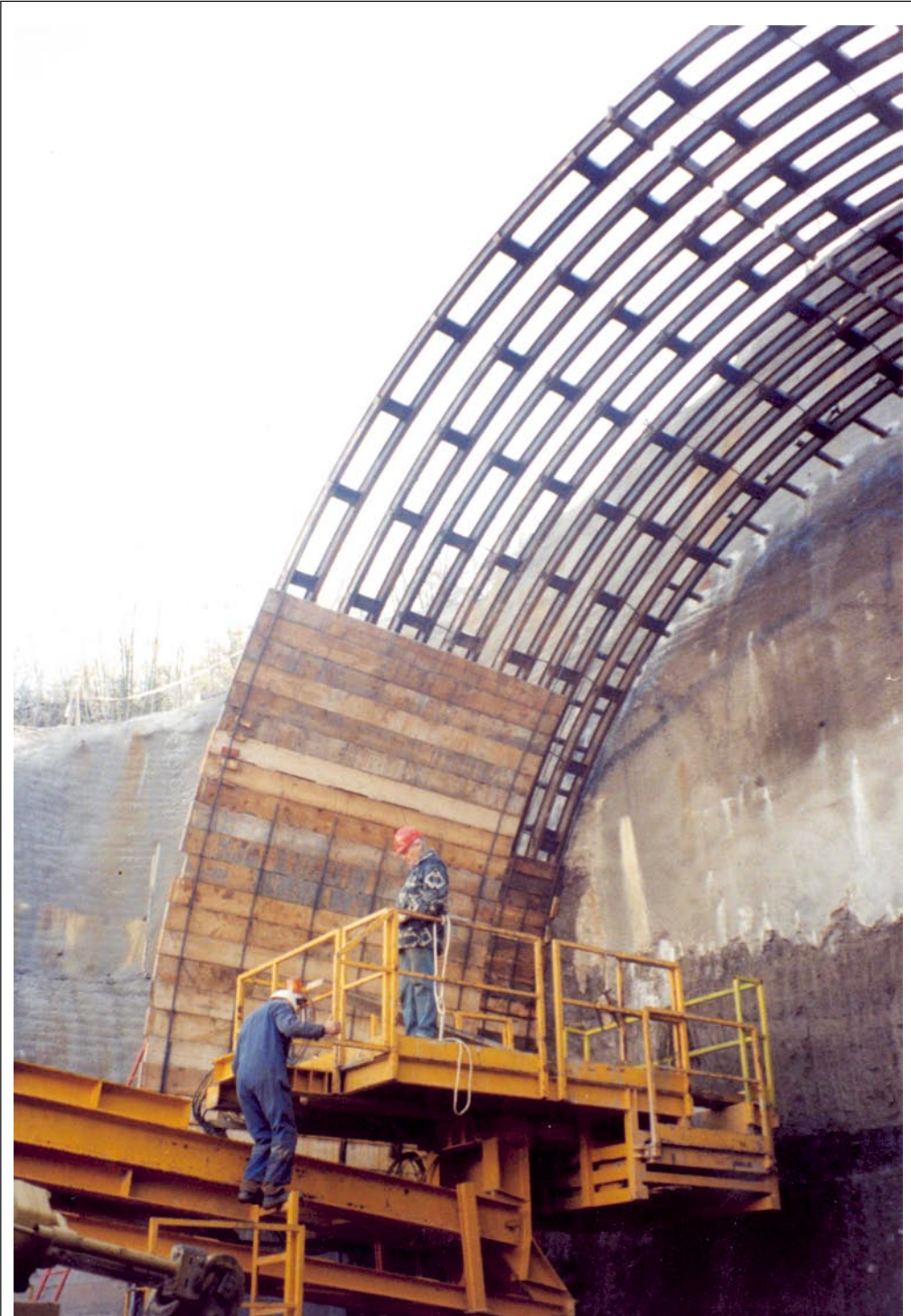
Macchia Piana Tunnel. Preparing the excavation scaffolding for the north portal
