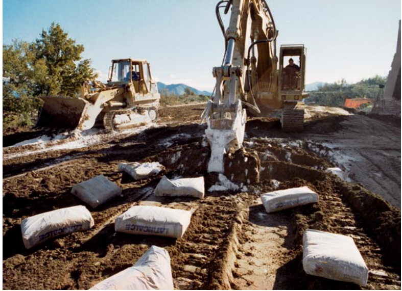
Piccilli 1 Tunnel: treatment of the ground with lime
