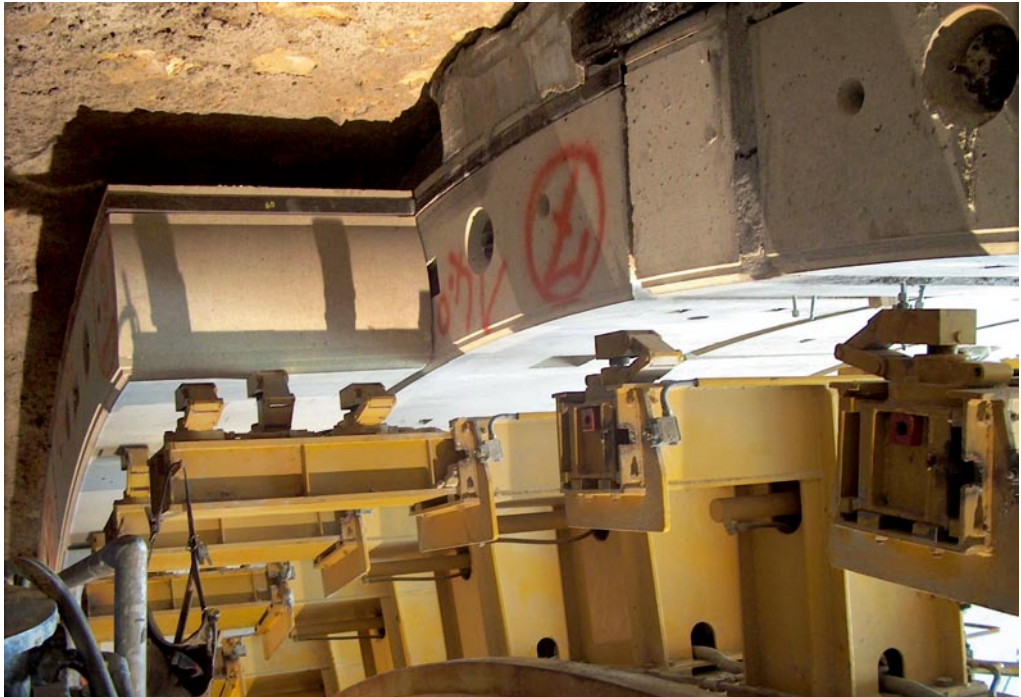
Fig. G.17 Erection of the prefabricated lining segments in prestressed r.c.
