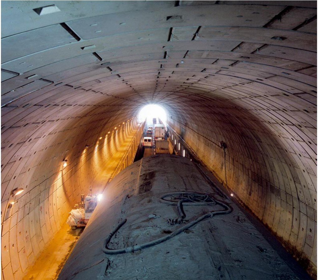
Fig. G.18 View of the widened tunnel
