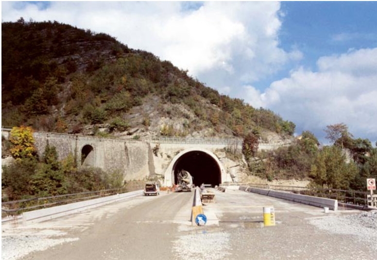
Scheggianico Tunnel. South tunnel under the state road (ground: Marly-Sandy formation)
