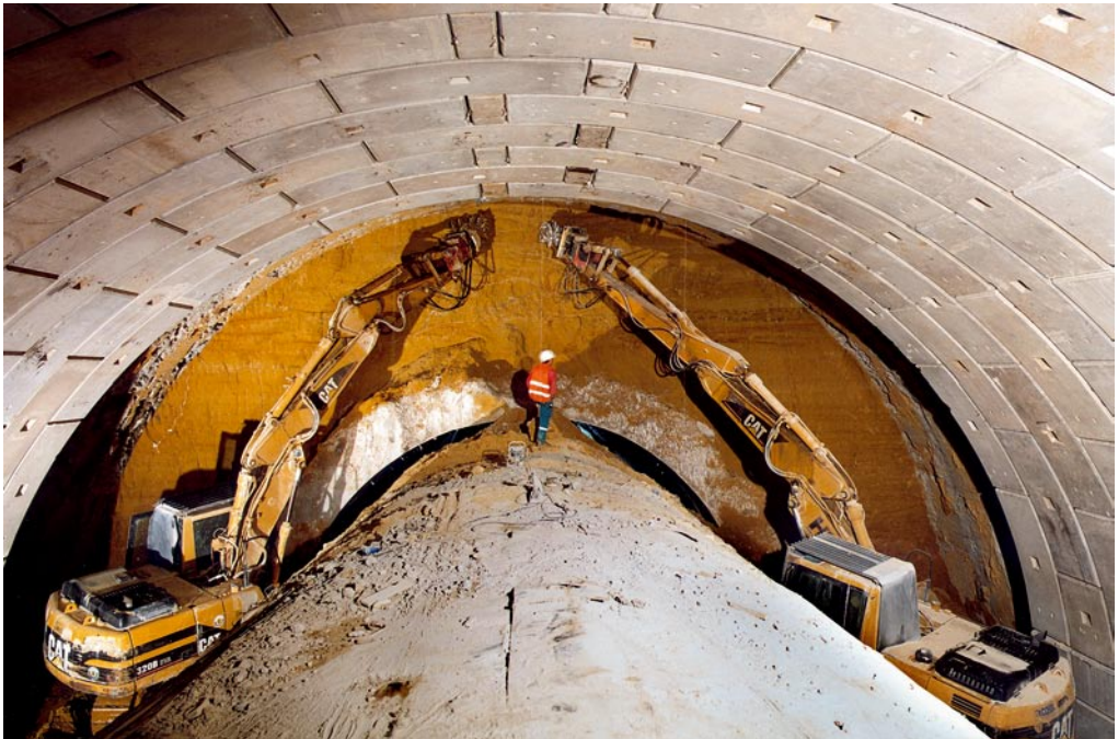
Fig. G.15 The widening face during demolition
