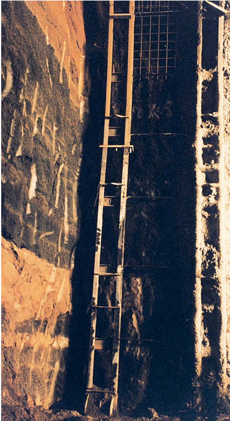
Galleria Colli Albani. Detail of a rib next to the face
