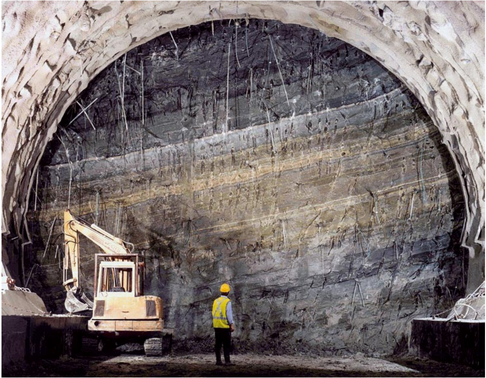
Fig. C.9 Reinforcement of the core-face by means of fibre glass structural elements
