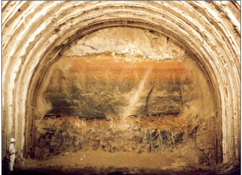
Colli Albani Tunnel. A typical face running through vulcanites, overburden: ~ 55 m
