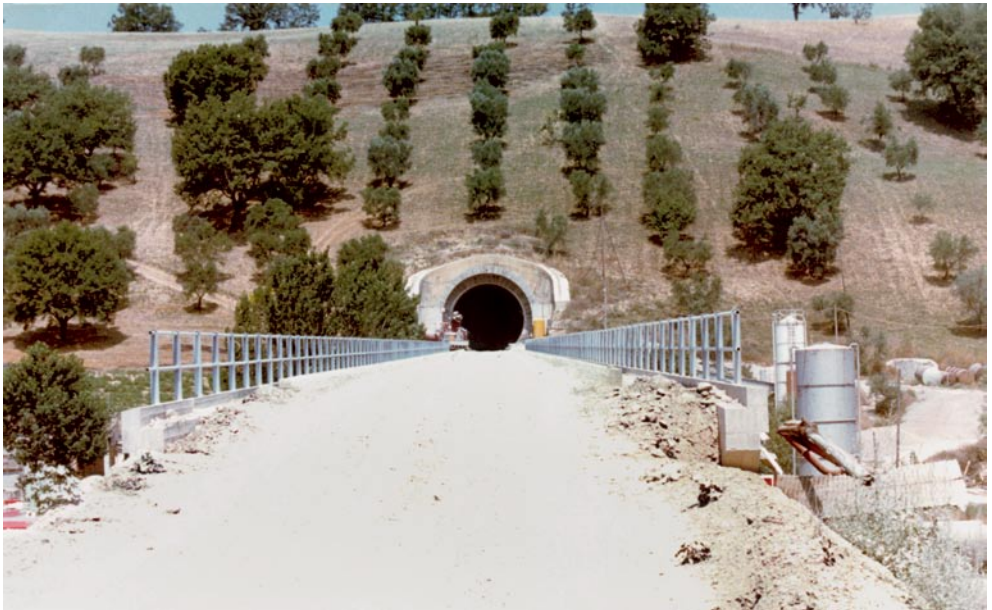
The same portal as above, seen from the front
