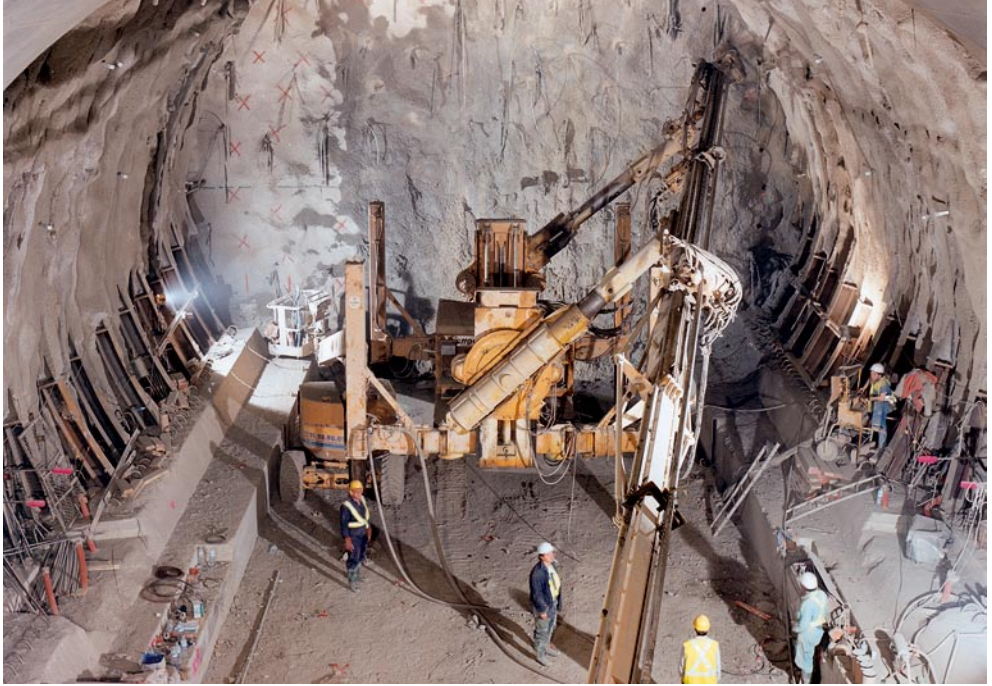
Fig. C.7 Reinforcement of the advance core
