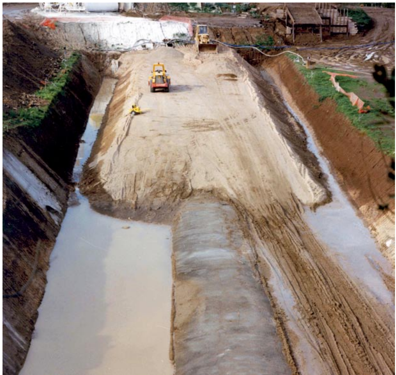
Piccilli 2 Tunnel: backfill with stabilised ground and compaction
