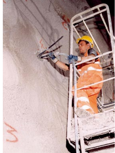
Raticosa Tunnel. Two moments in the reinforcement of the advance core using fibre glass structural elements. Drilling and insertion (left); cementation (right)
