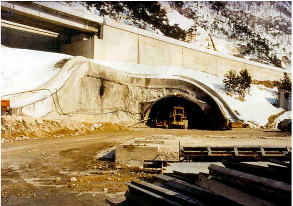
Fig. F.4 The portal of the same tunnel during excavation works
