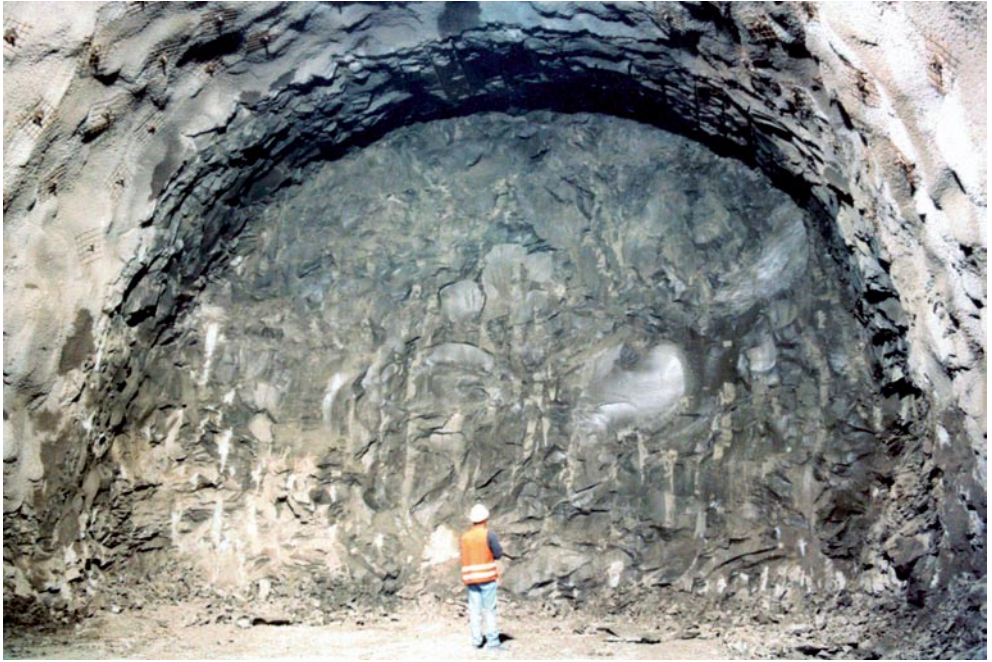
Monte Bibele Tunnel. View of the face while tunnelling through the Bismantova Marls, overburden: ~ 40 m)
