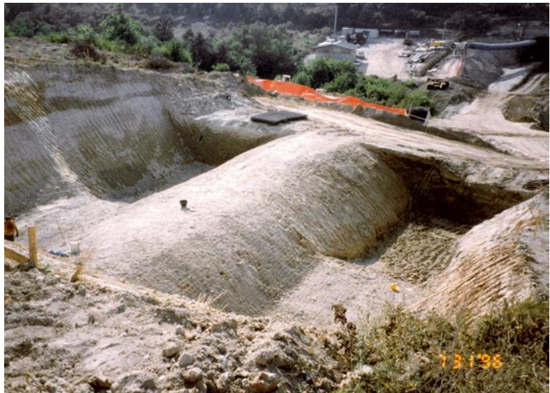
Piccilli 1 Tunnel: shaping the extrados of the future tunnel
