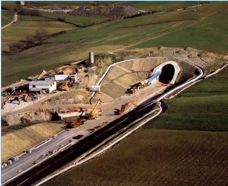
Colle Pece Tunnel. North portal
