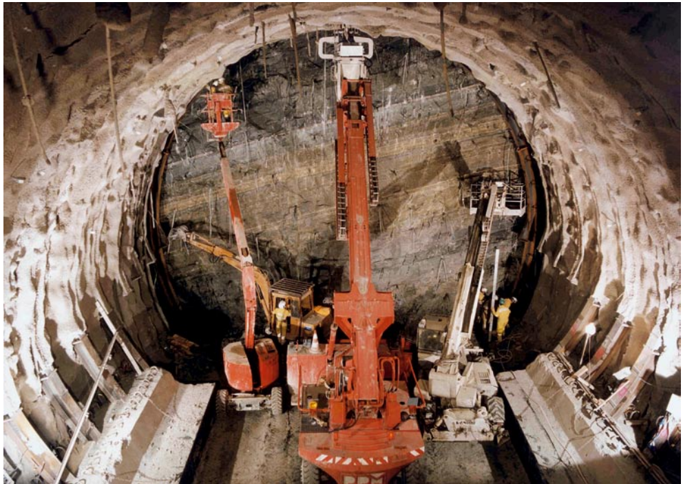
Fig. C.8 Placing of steel ribs
