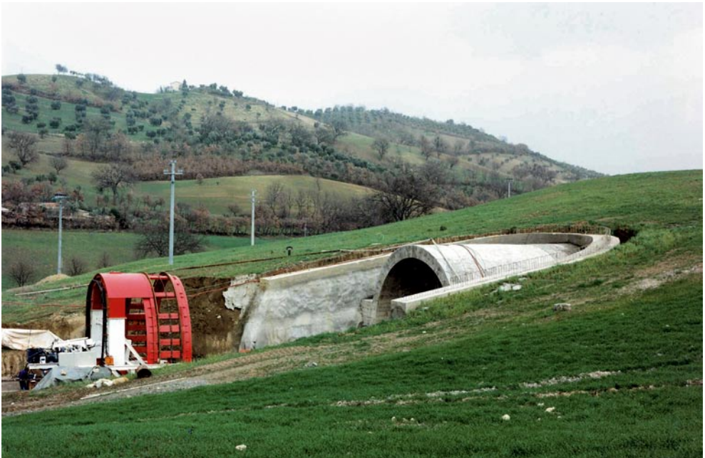
The same portal as above: notice the extremely shallow overburden of the tunnel and the way it fits perfectly into the landscape of the environment
