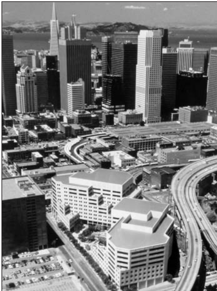
Left: 303 Second Street, San Francisco. The court was located on the top two floors of the foreground building from 1991 to 1999.
