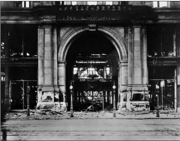
The damaged entrance to the Emporium Building, 825 Market Street, San Francisco, 1906. The court was located here during the great earthquake and fire.
