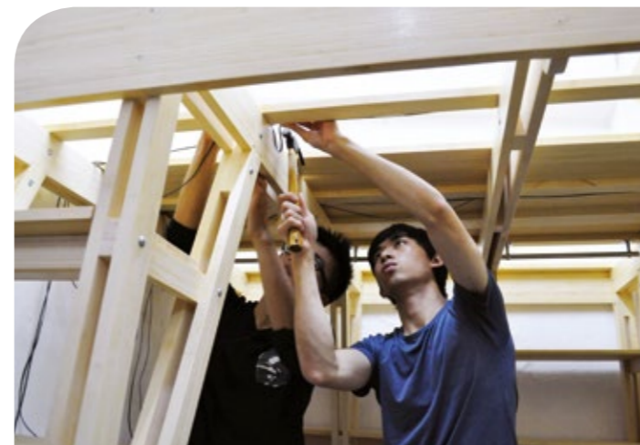
Students constructing the bunk bed.
