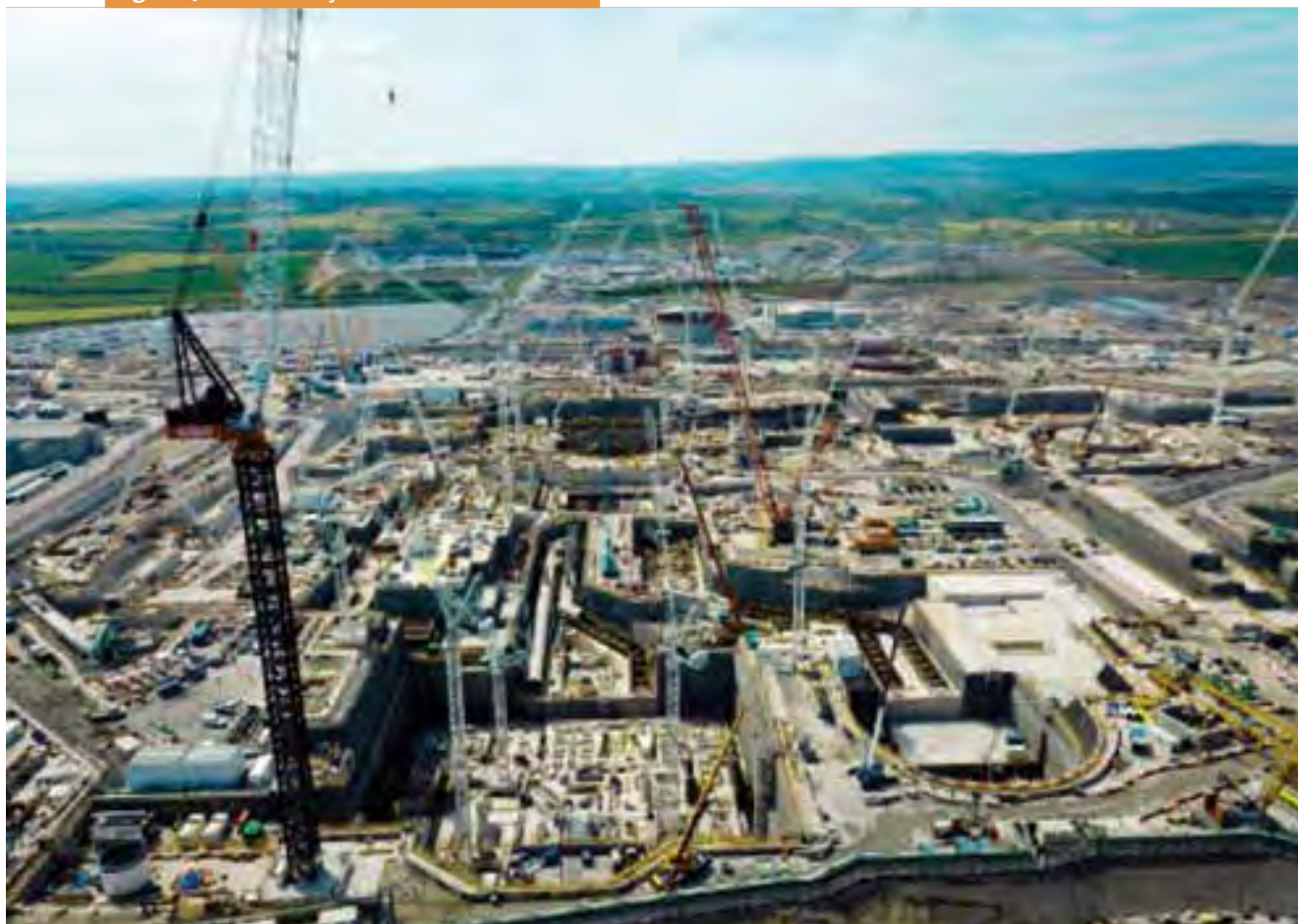
Figure 42 : The Hinkley Point C Construction Site
