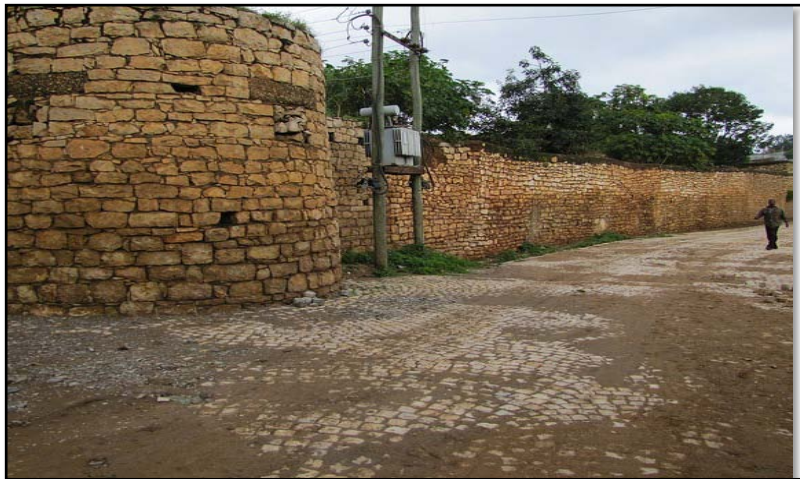
Photo 15:- A Section of Jugal Wall on the side of Badro Bari
