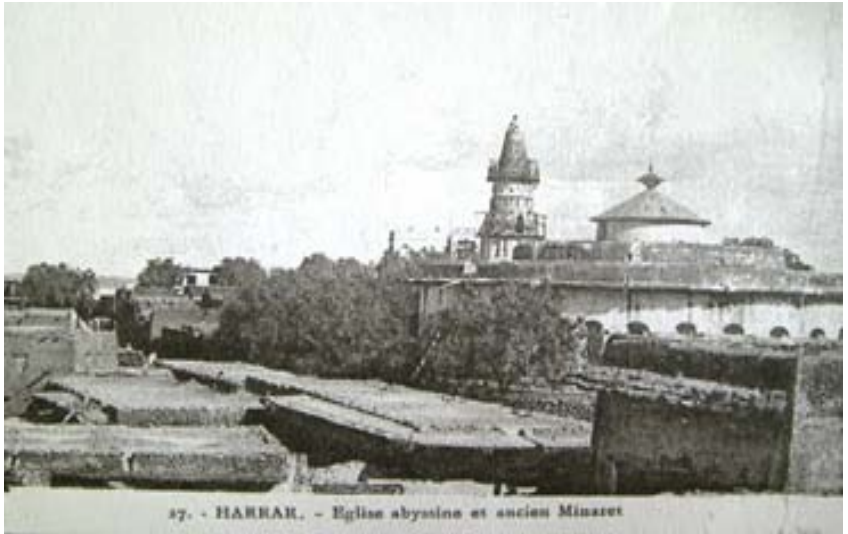
Photo 5:-The Sheikh Bazikh Mosque (under destruction) and the Dome of Medhane Alem Church (simultaneously in process of erection) – 1897
