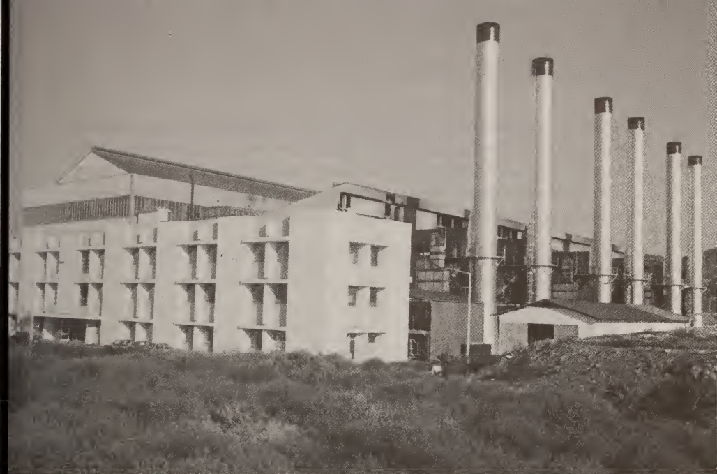
Dhekelia Power Plant Courtesy Embassy of Cyprus, Washington
