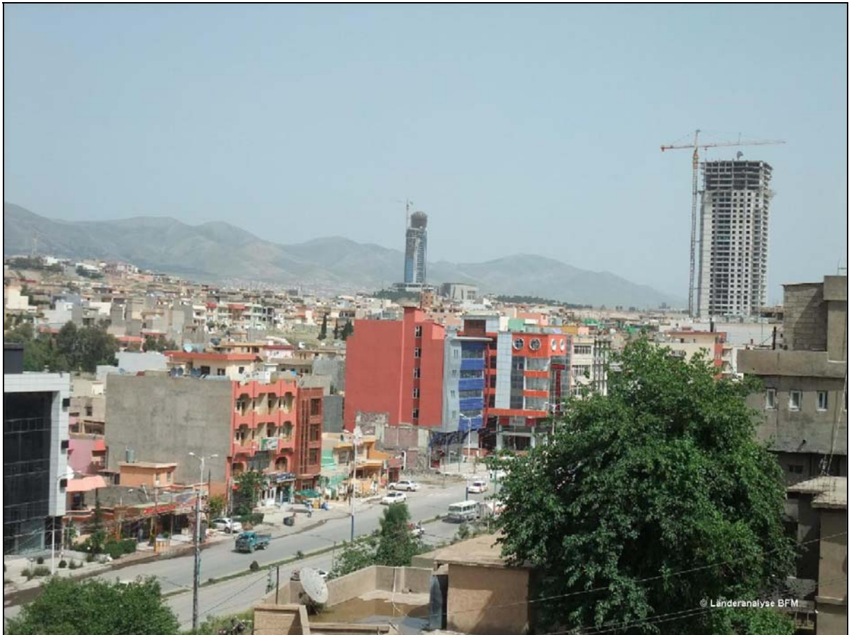
New skyscrapers under construction in Sulaymaniya.
