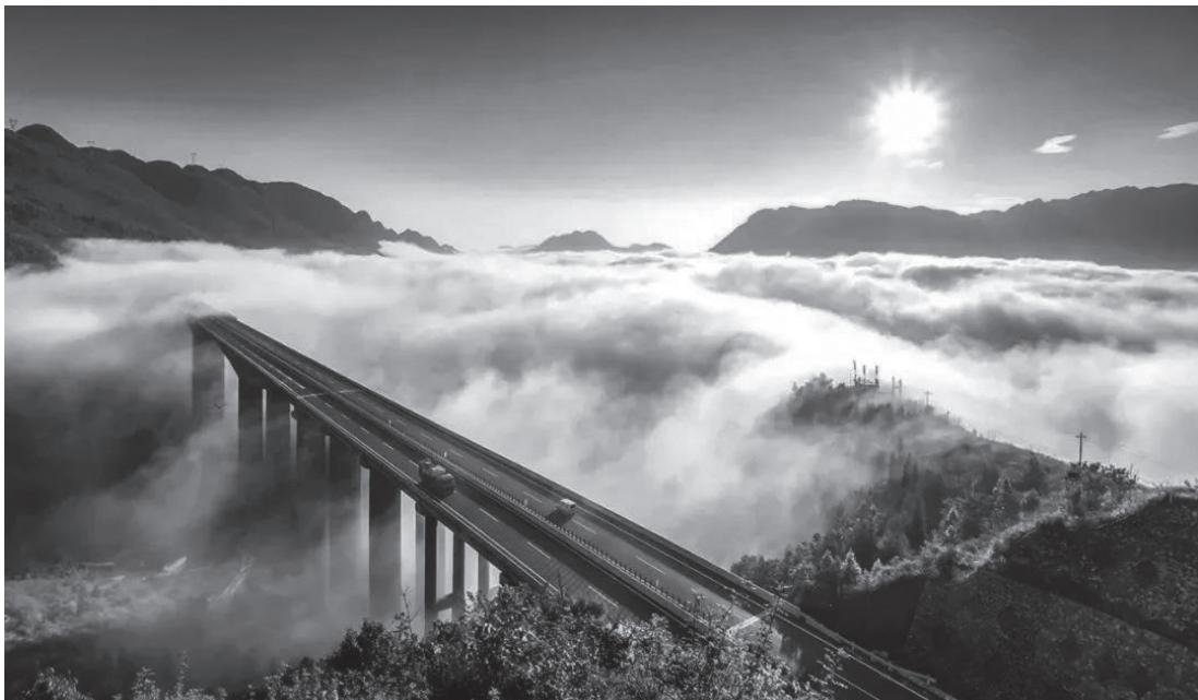
Picture: 3.3 He Zhang bridge, Biwei Highway, Guizhou Province.
