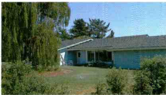
NICE HOME W/GREAT POOL $1,195,000 Santa Ynez. 3bd/2.5ba on cul-de-sac on almost 1 acre. Large living area, tile floors, rock fireplace. French doors, patio. Room for horses.
