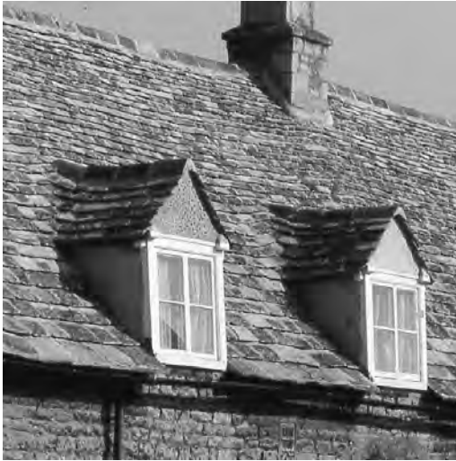
Fig. 4 Easton on the Hill (Northants.). Eaves dormer windows on an 18th-century cottage. Photograph, author
