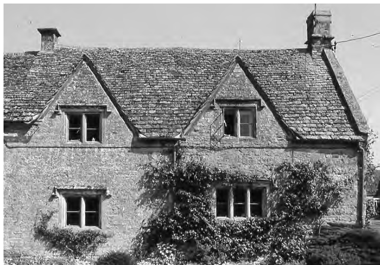
Fig. 3 Bledington (Glos.). First-floor windows in Cotswold gables breaking the eaves line. Photograph, author
