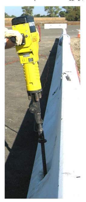
Figure 7-7. Stake Installation
