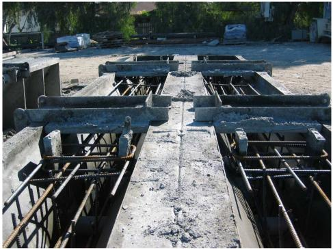
Figure 2-2. K-rail Rebar Placement
