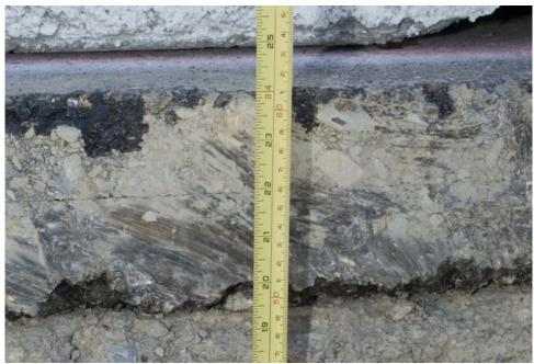
Figure 2-1. Asphalt Concrete Thickness
