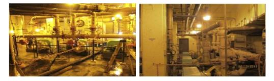
Secondary sludge is pumped from the clarifiers to a sludge storage tank prior to sludge thickening. The sludge pumping system includes three (3) Wemco vortex type sludge pumps.
