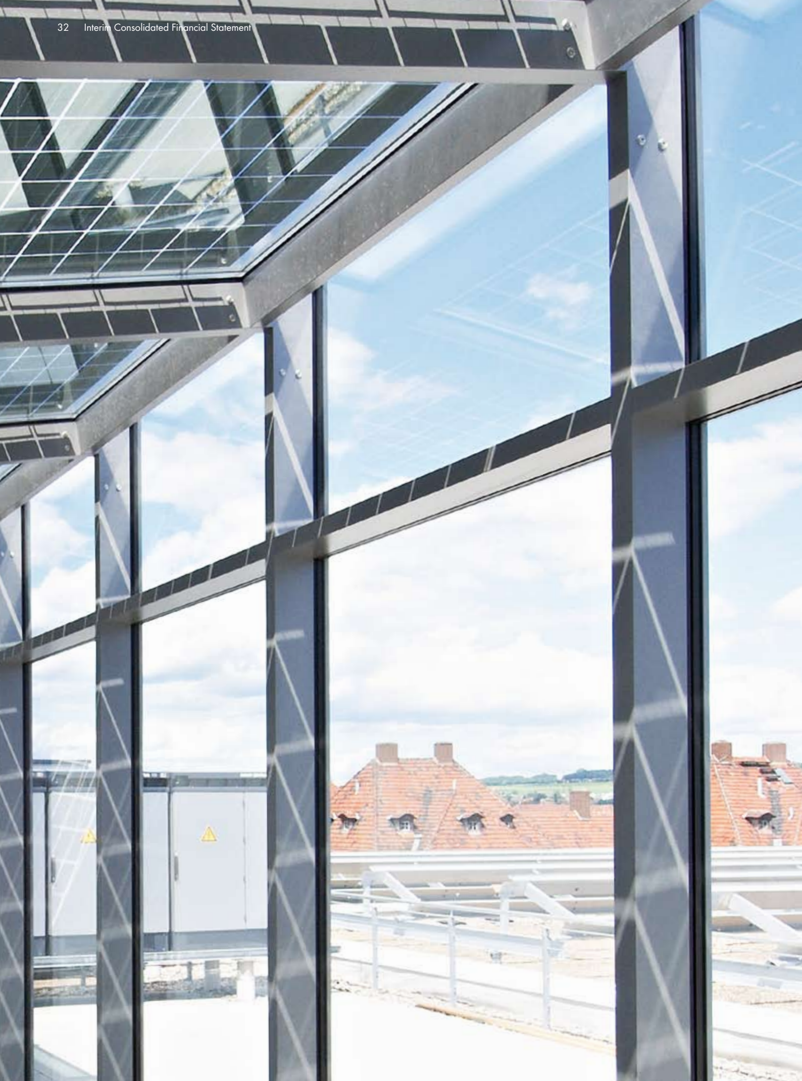
The integrated PV system with a power of around 1.1 megawatt on the CO 2 -neutral inverter factory is partially equipped with Sunny Central 100 Outdoor inverters.
