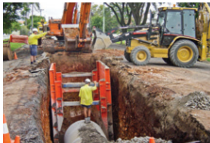
Construction of stormwater infrastructure
