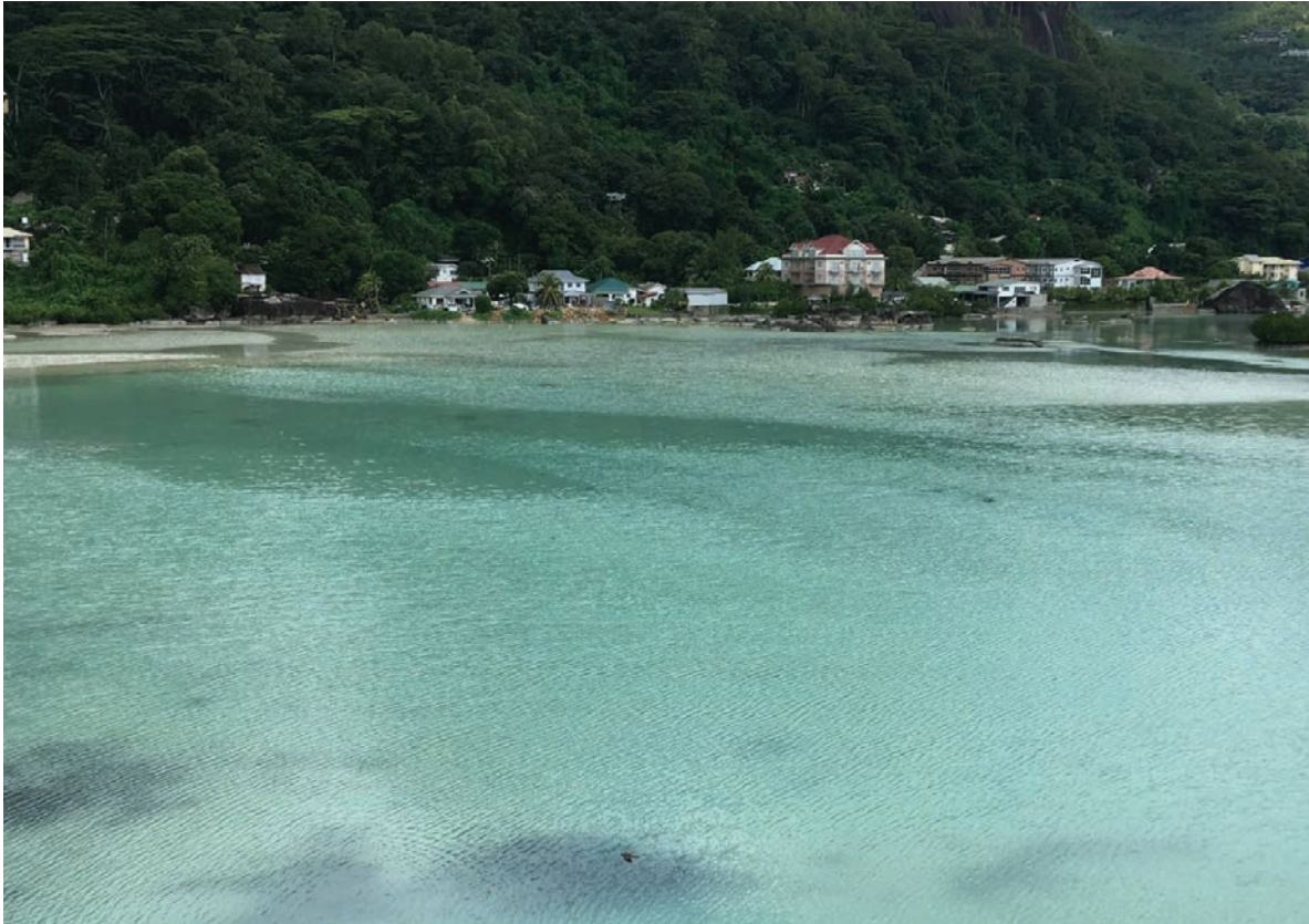
In 2019, as part of an ongoing transition to renewable energy in the Seychelles, our climate initiative partnered with the local government and Public Utilities Corporation to implement a marine floating solar power plant in Providence Lagoon on Mahé Island.
