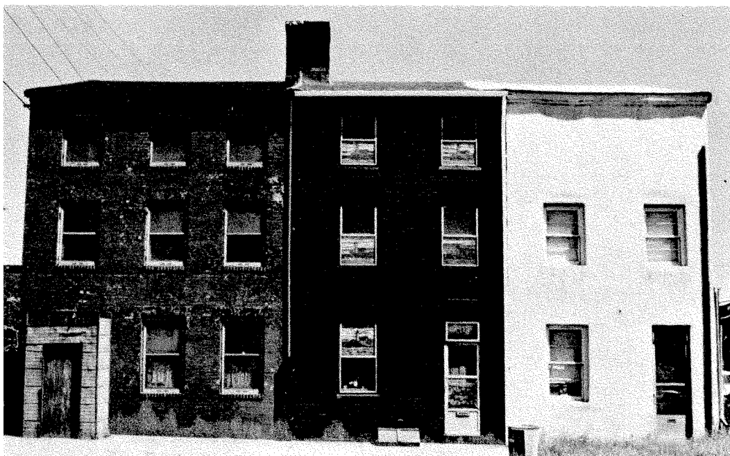
Last three houses of Copper Row
