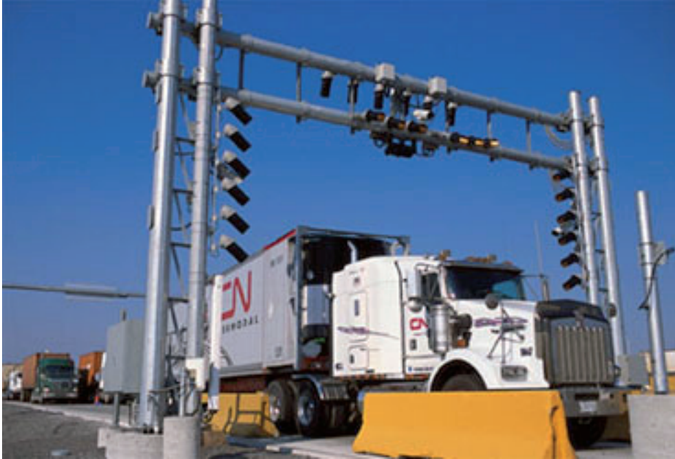
Figure 54. Automated Gate Systems at CN intermodal facility in Brampton
