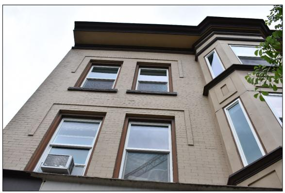
Fig. 11 – East facade, detail of masonry window hoods and bay windows.
