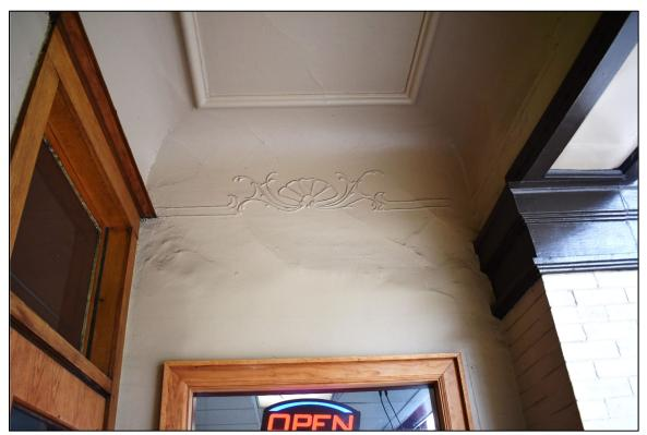
Fig. 19 – North facade, detail of E Denny Way building entrance, showing coved ceiling and plasterwork.
