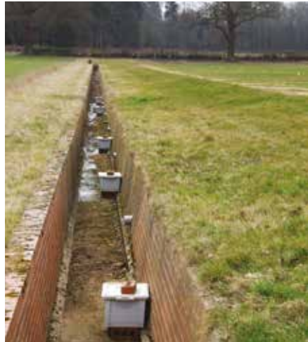
Drain outlets at eastern end of Broadbalk, 2010
