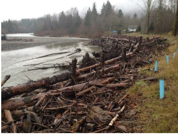
Figure 41: Complex timber revetment (photo credit: Tim Abbe, USBR and ERDC 2016).
