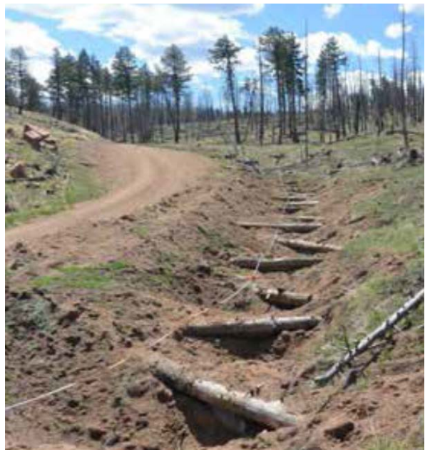
Figure 66: Log "rock and roll" channel in the Trail Creek watershed, Colorado (USFS 2015).
