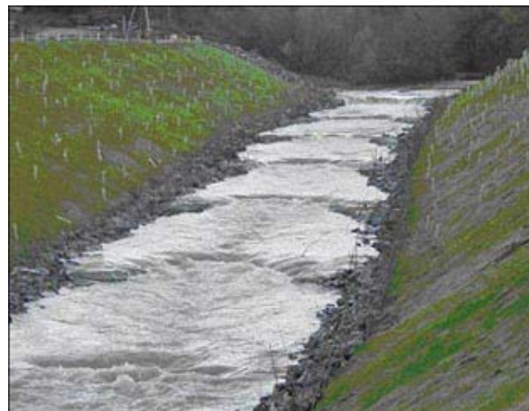
Figure 47: Pool and weir fishway.
