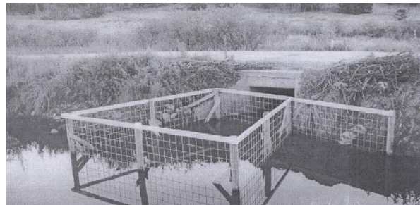
Figure 50: Beaver deceiver (Brown et al. 2001).
