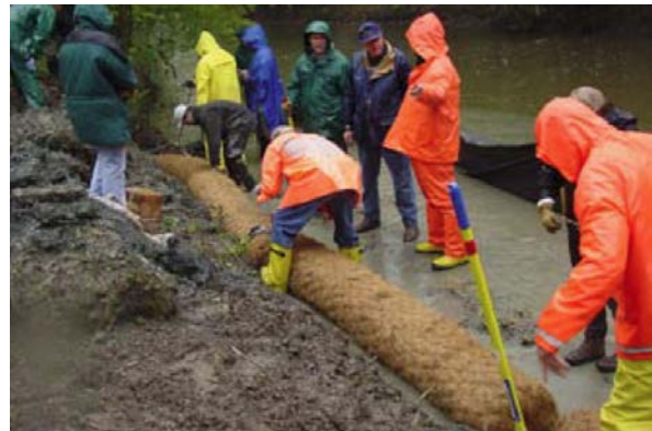
Figure 58: Installation of coir fascines (NRCS 2007, TS14I).
