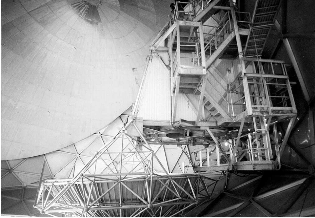
Figure 16. A view inside the Gregorian showing part of the secondary reflector, the tertiary (bottom) and the feed tower.
