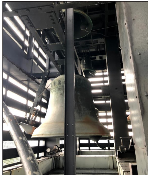
Figure 86. Rust staining on bell, photo by author
