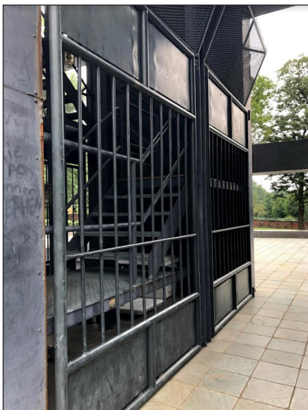
Figure 68. Exterior of Stair Cage (2019), photo by author
