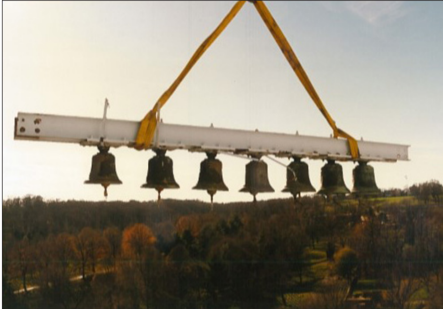
Figure 32. Bells being removed in 1995 for rehabilitation work, GWMP archives
