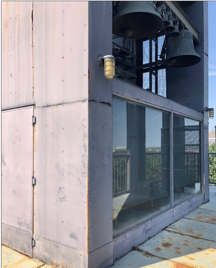
Figure 55. East Elevation of clavier playing chamber, photo by author
