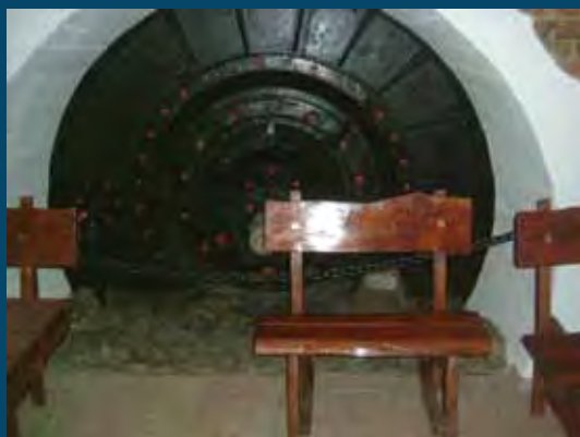
HE pastate Inside powerhouse
