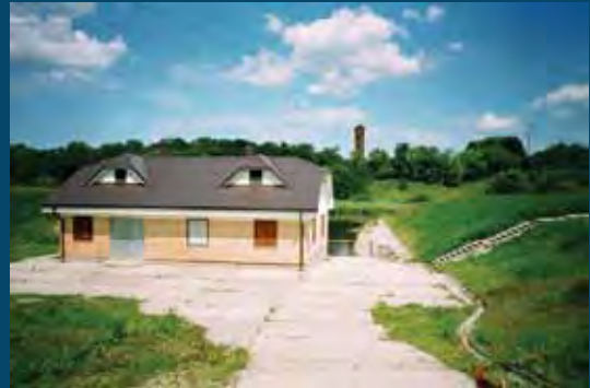
HE pastatas Powerhouse
