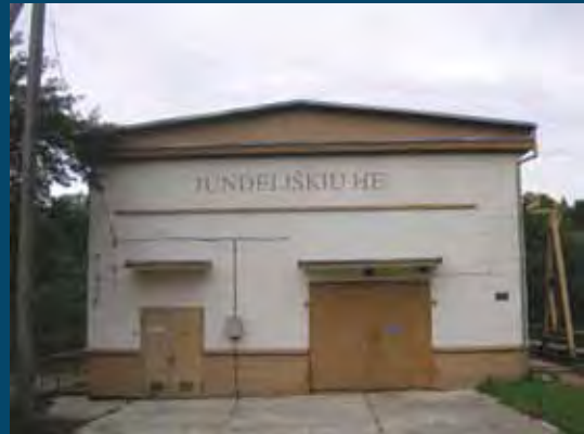
HE pastatas Powerhouse
