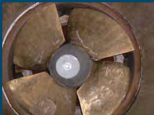
Hidroturbina remonto metu Hydroturbine during repair
