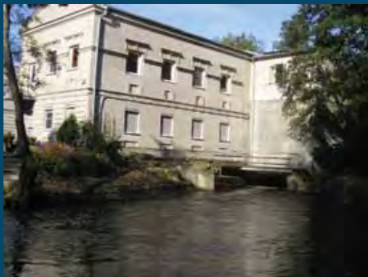
HE pastatas Powerhouse
