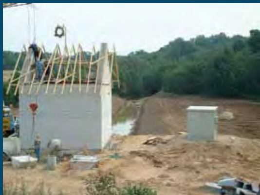
HE pastatas statybos metu Powerhouse during construction
