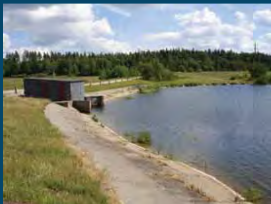
HE vandens ėmykla Water inlet structure
