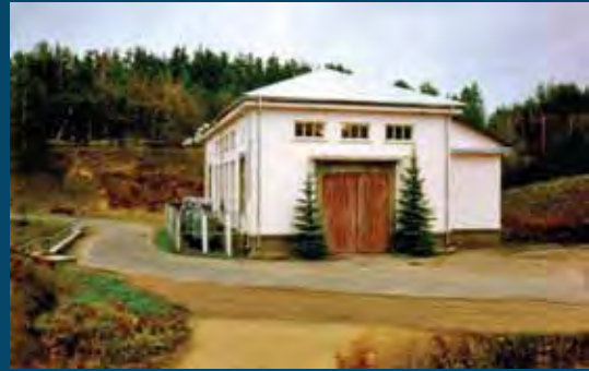
HE pastatas Powerhouse
