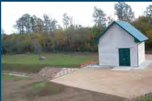
HE pastatas Powerhouse
