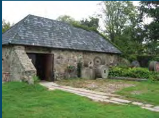
HE pastatas Powerhouse
