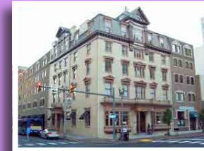
6 COLONIAL THEATRE ▶ 3rd and Market Streets ▶ Style: Greek Revival ▶ Designated: 1982
