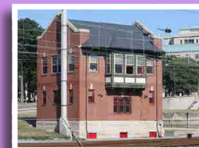
12 HARRIS SWITCH TOWER ▶ 637 Walnut Street ▶ Style: Georgian ▶ Designated: 1994
