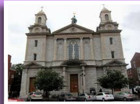
5 CATHEDRAL OF SAINT PATRICK ▶ 219 South Front Street ▶ Style: Georgian ▶ Designated: 1975
