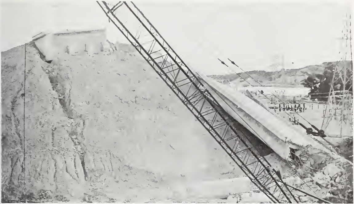
Figure 7.15 East abutment of IS 210/5 Separation and Overhead structure.
