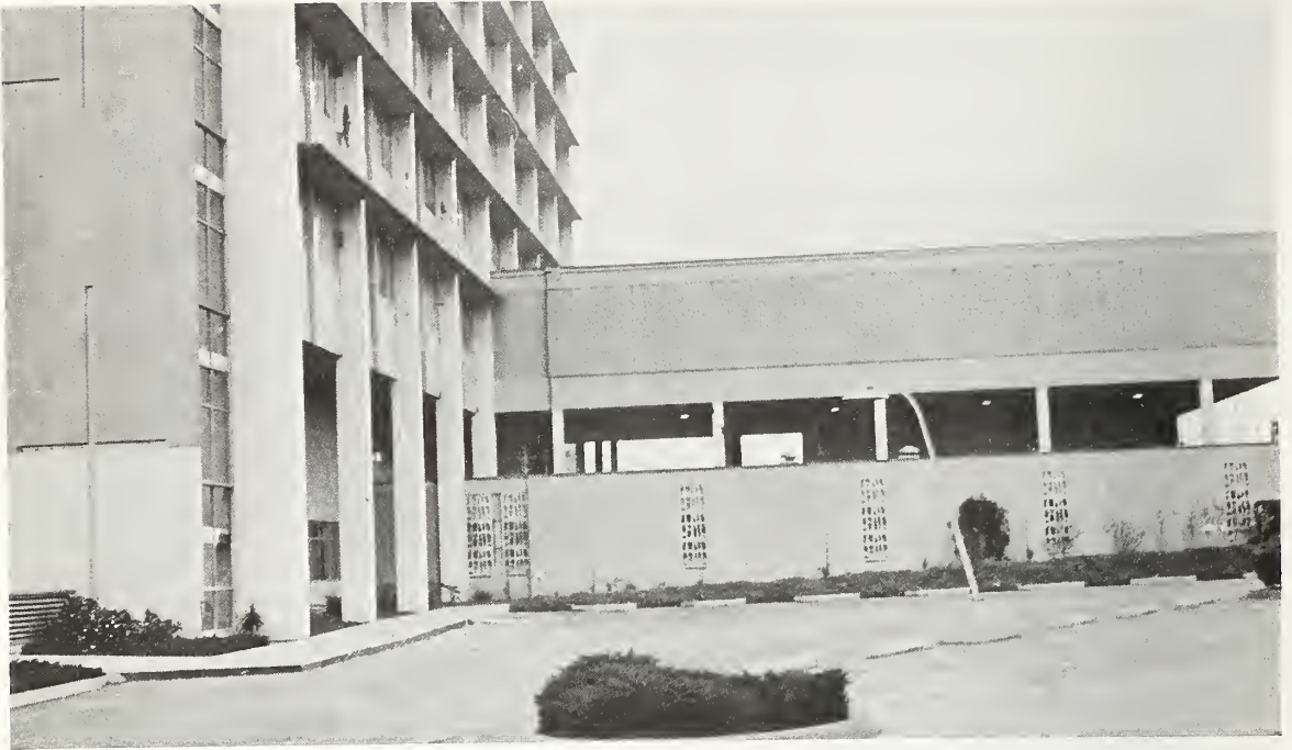
Figure 5.73 East elevation of three-story north wing. The east row of the second-story columns are shown in figure 5.74.
