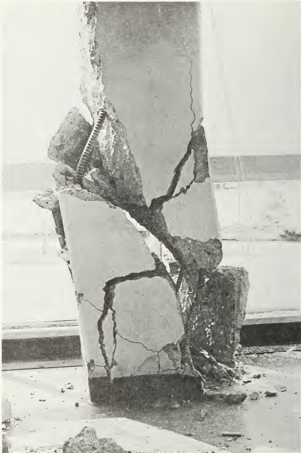
Figure 5.64 Reinforced concrete column at the west end of the third story.
