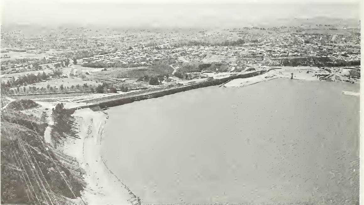
Figure 4.5 Lower San Fernando Dam and endangered residential area.
