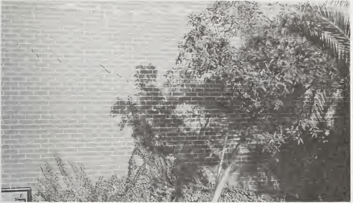
Figure 5.80 Reinforced brick masonry shear wall at west end of south section.
