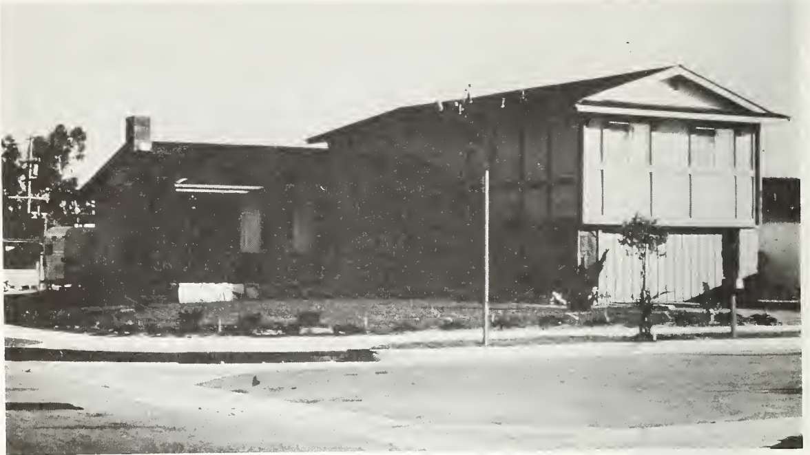
Figure 5.158 Undamaged split-level residence at Fenton Avenue and Tyler Street.
