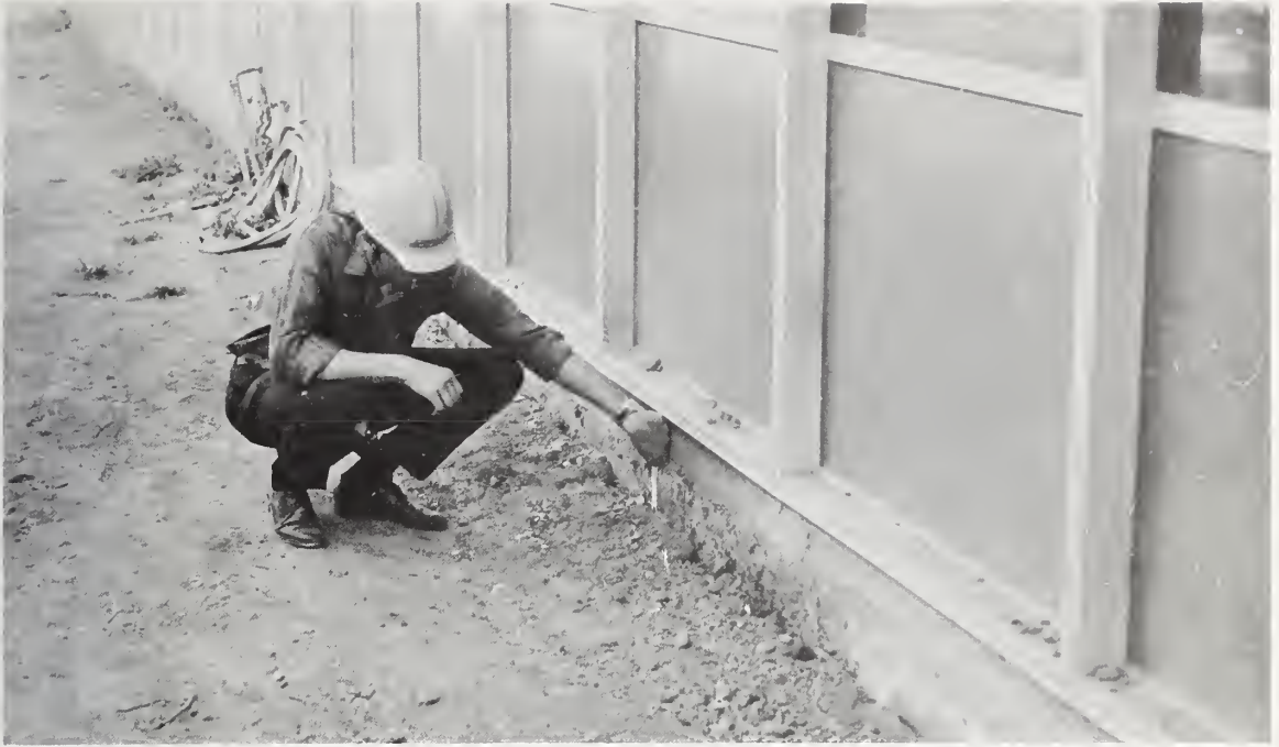
Figure 5.86 Relative movement between north section and ground.
