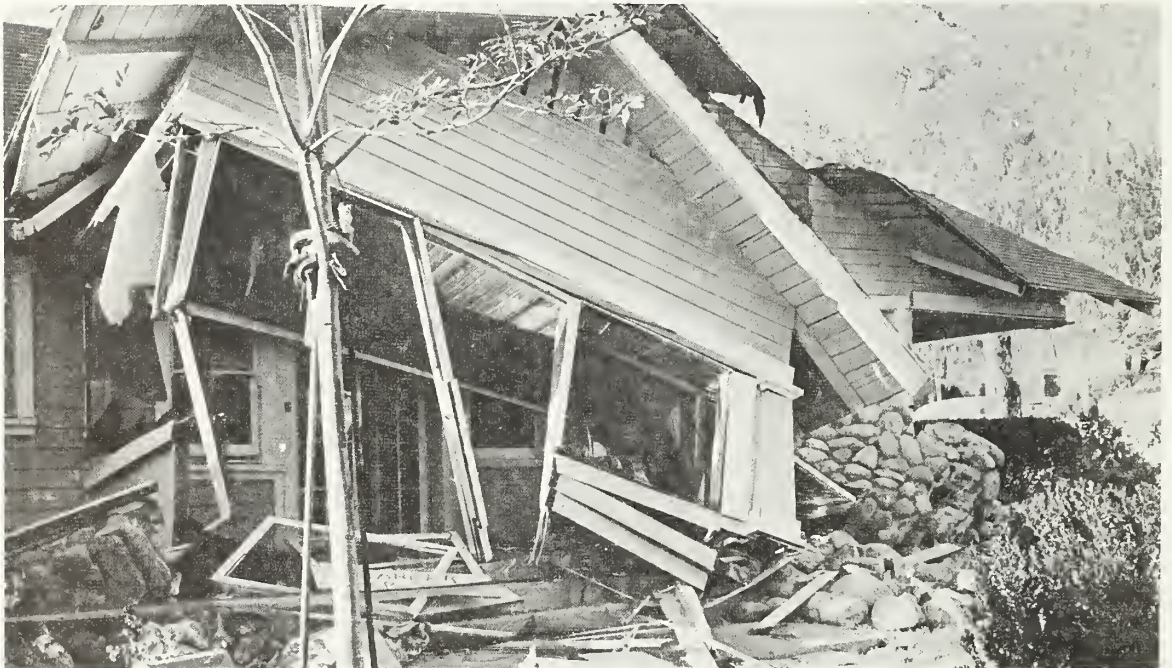
Figure 5.167 Destroyed wood-frame house.
