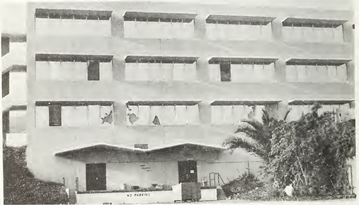
Figure 5.79 South elevation of center section.
