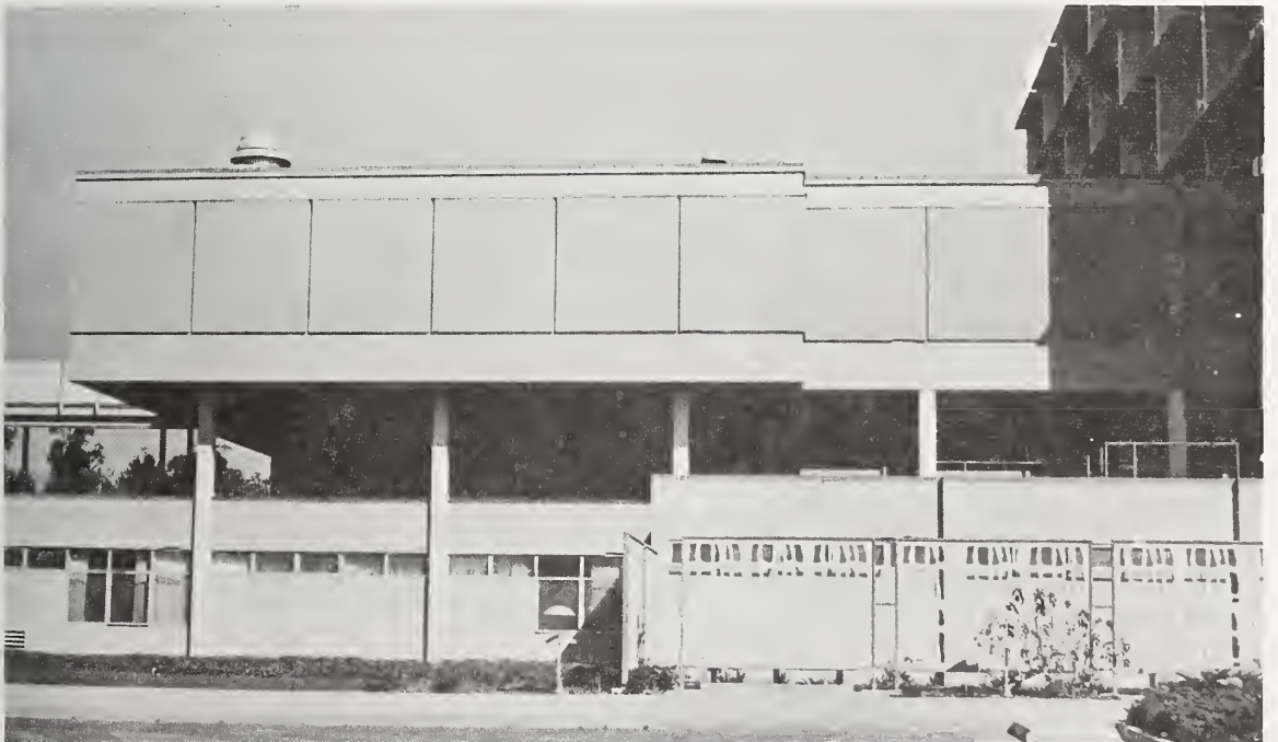
Figure 5.72 West elevation of North Wing.
