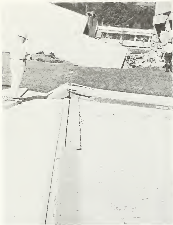
Figure 5.17 Compression ridge (arrow) on the north side of the main building.
