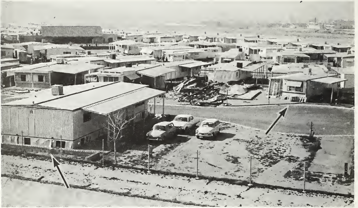
Figure 5.174 Mobile home park located along Sierra Highway 14 in Newhall. At the center of the figure are the remains of a home which was completely destroyed by fire. Note damaged metal curtain walls around the bases of the mobile homes (arrows).
