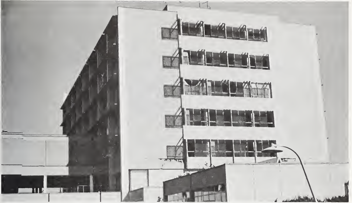
Figure 5.62 West elevation of tower.
