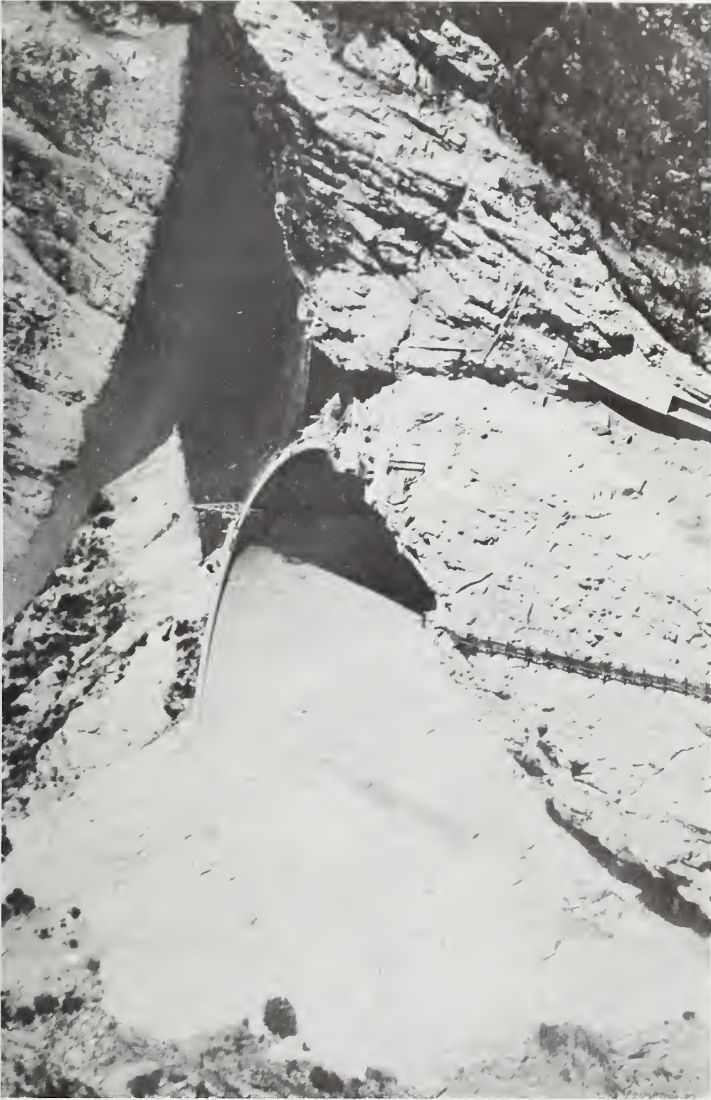
Figure 8.26 Pacoima Dam, a 370-ft high concrete-arch dam, built in 1928.
