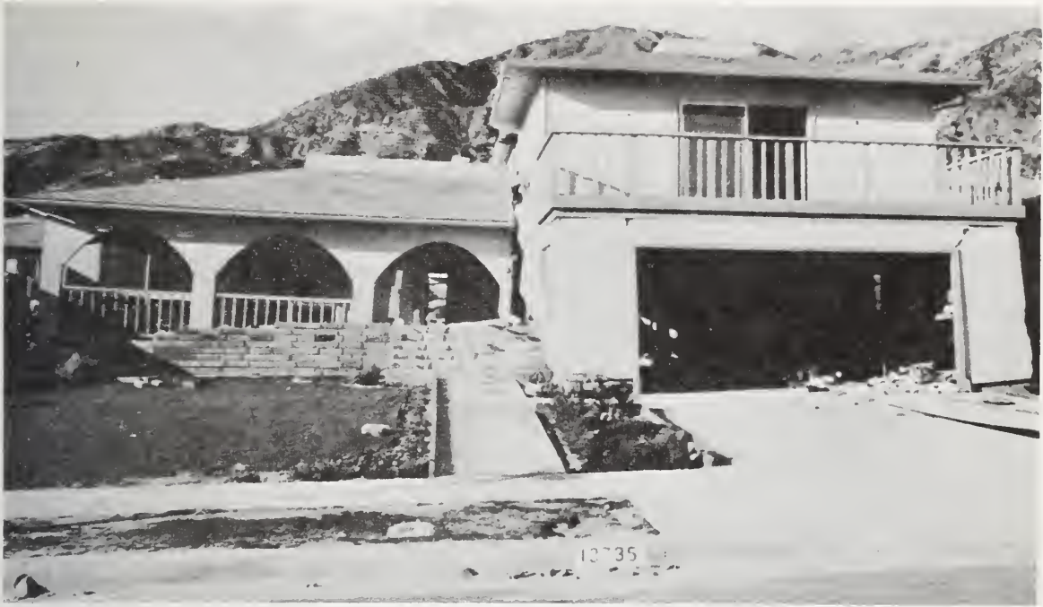
Figure 5.160 Damaged split-level residence at Aldergrove Street and Leedy Avenue.
