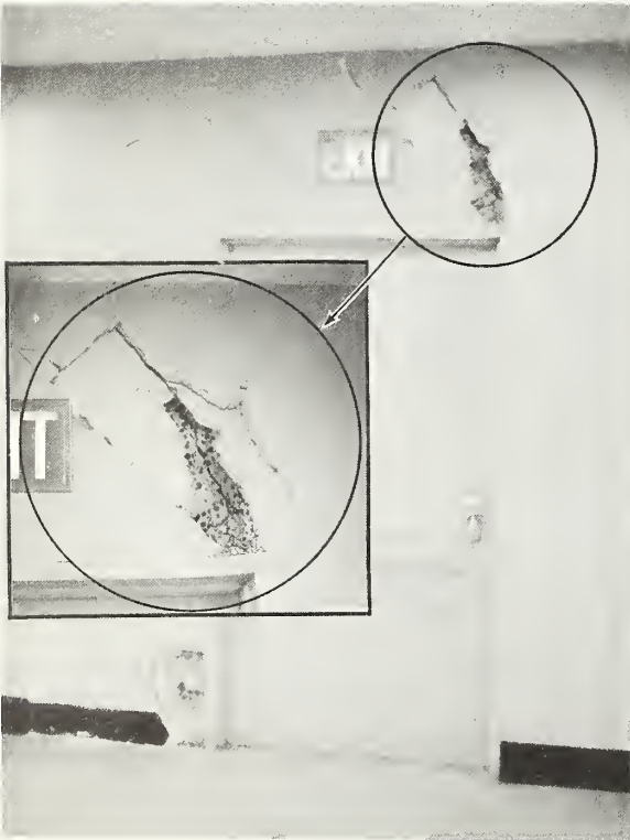
Figure 5.96 Crushed reinforced concrete elevator shaft on the first floor. Note the exposed reinforcing steel. (See fig. 5.94, location 1).
