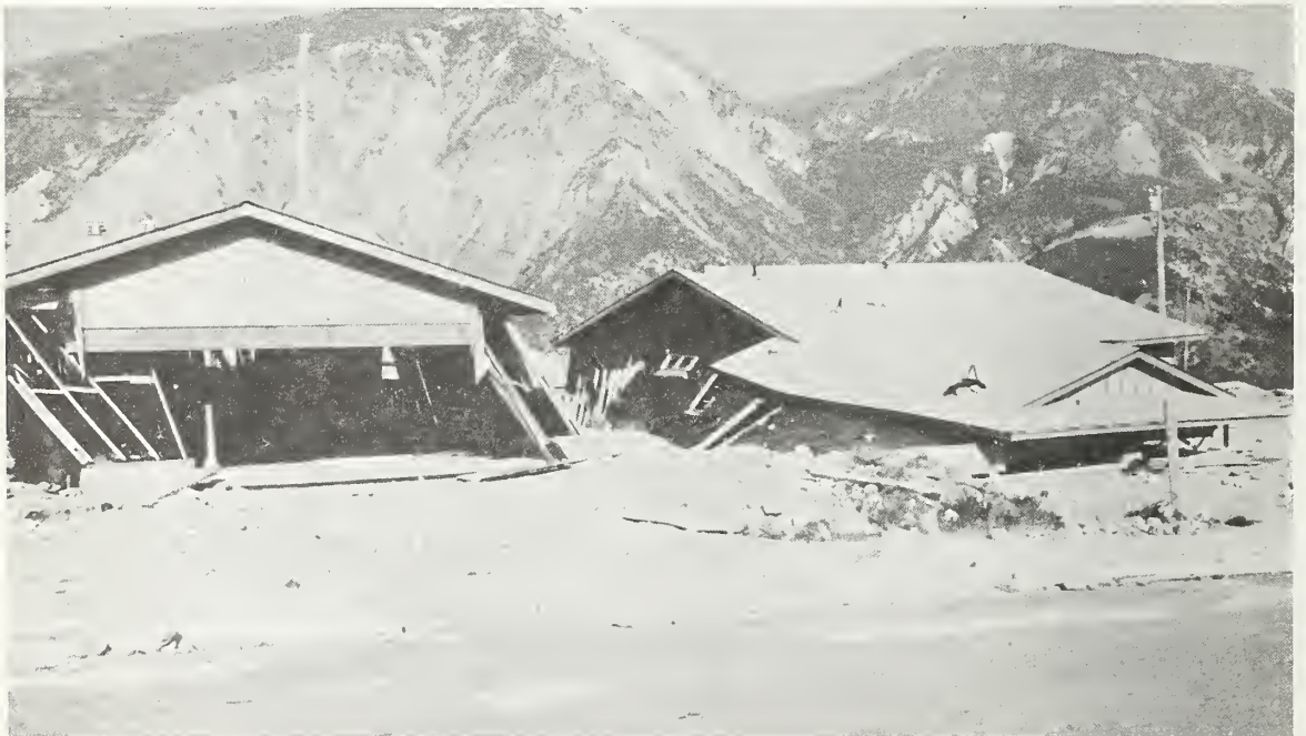
Figure 5.169 Partially collapsed houses under construction.
