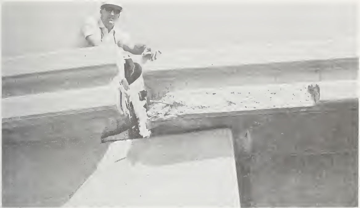
Figure 7.30 Longitudinal and transverse movement of cast-in-place box girders with respect to abutment sections.
