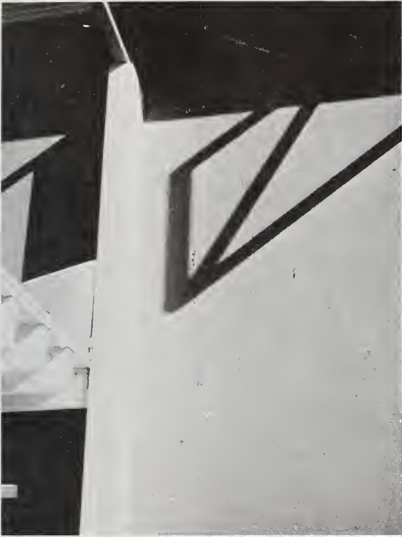
Figure 6.47 Clerestory windows of gymnasium fell out and bracing rods stretched, Los Angeles County Juvenile Facility.
