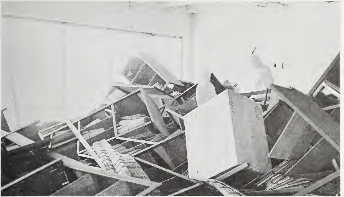
Figure 5.71 Shaking caused shelves to overturn on the seventh floor.
