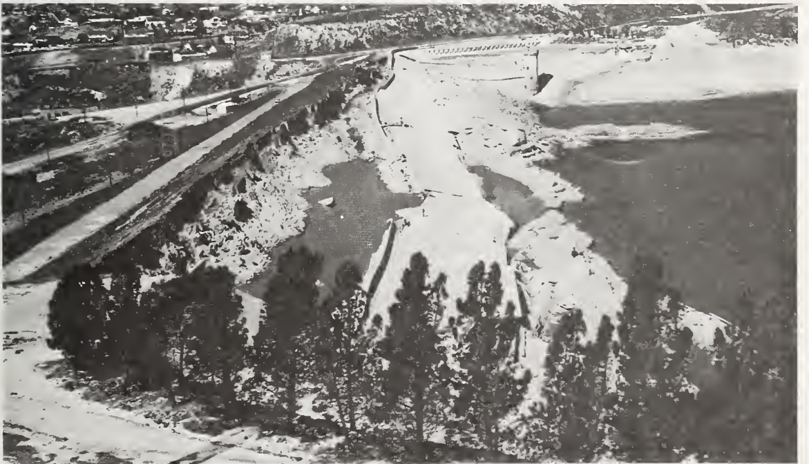
Figure 4.7 Collapsed liner of Lower San Fernando Dam.
