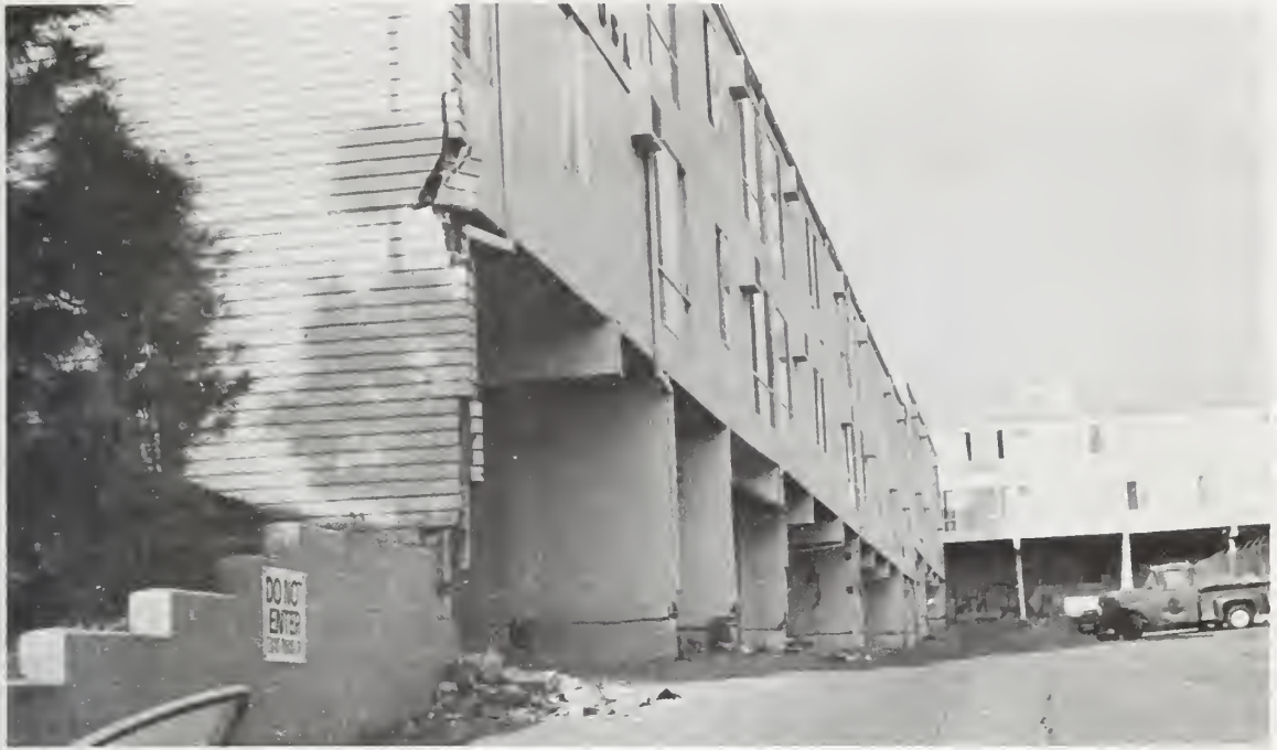
Figure 5.170 Rear view of damaged three-story "Friday USA" apartment building.
