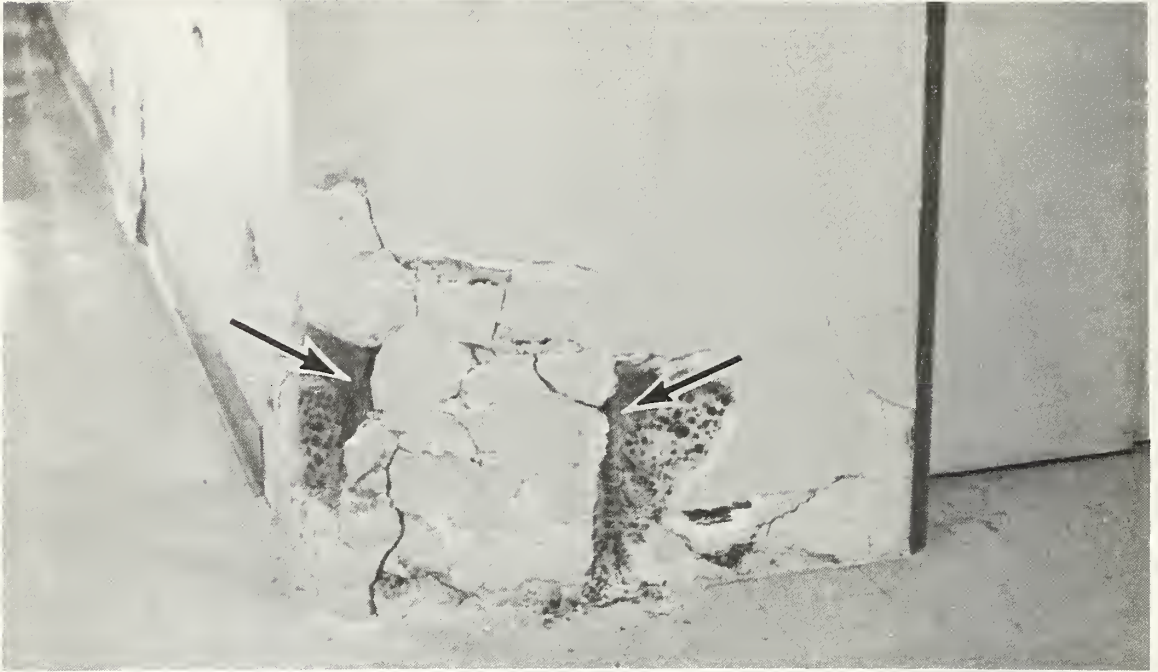
Figure 5.96 Crushed reinforced concrete elevator shaft on the first floor. Note the exposed reinforcing steel. (See fig. 5.94, location 1).
