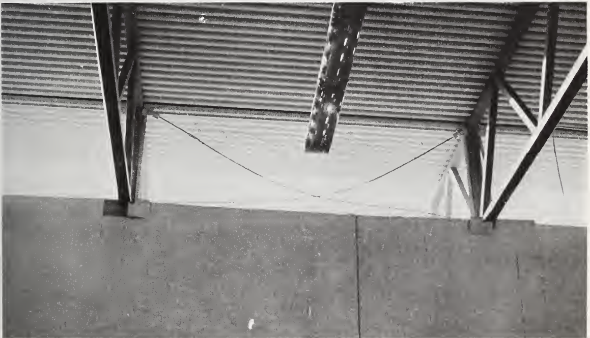
Figure 6.47 Clerestory windows of gymnasium fell out and bracing rods stretched, Los Angeles County Juvenile Facility.
