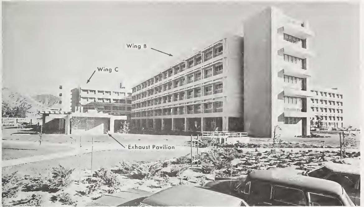
Figure 5.32 Typical stair tower before the earthquake.
