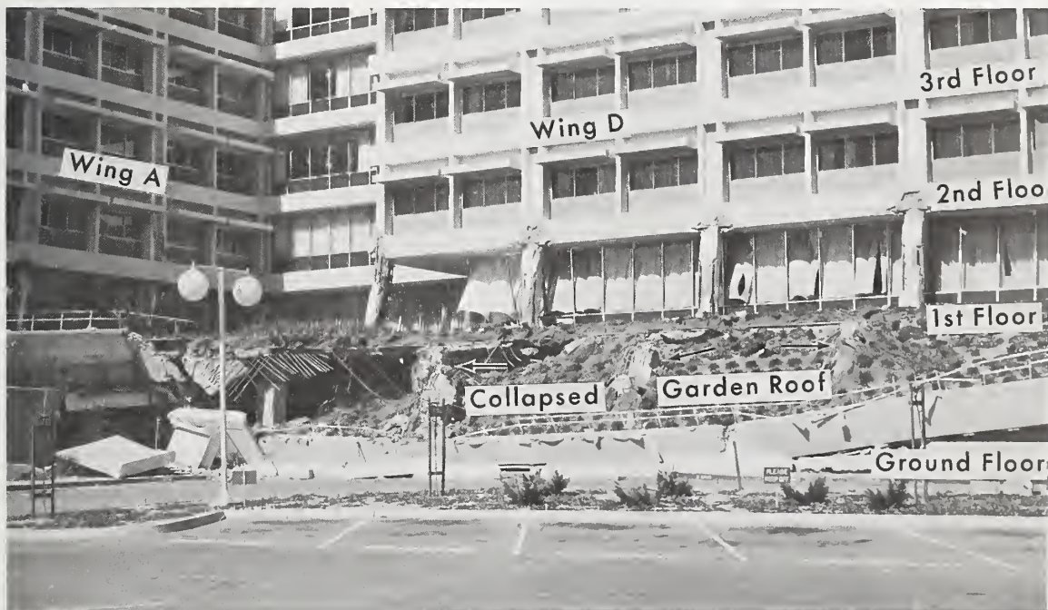
Figure 5.23 South face of Wing D. Note that the bulk of major damage suffered by the building is limited to the ground, first, and second floors.
