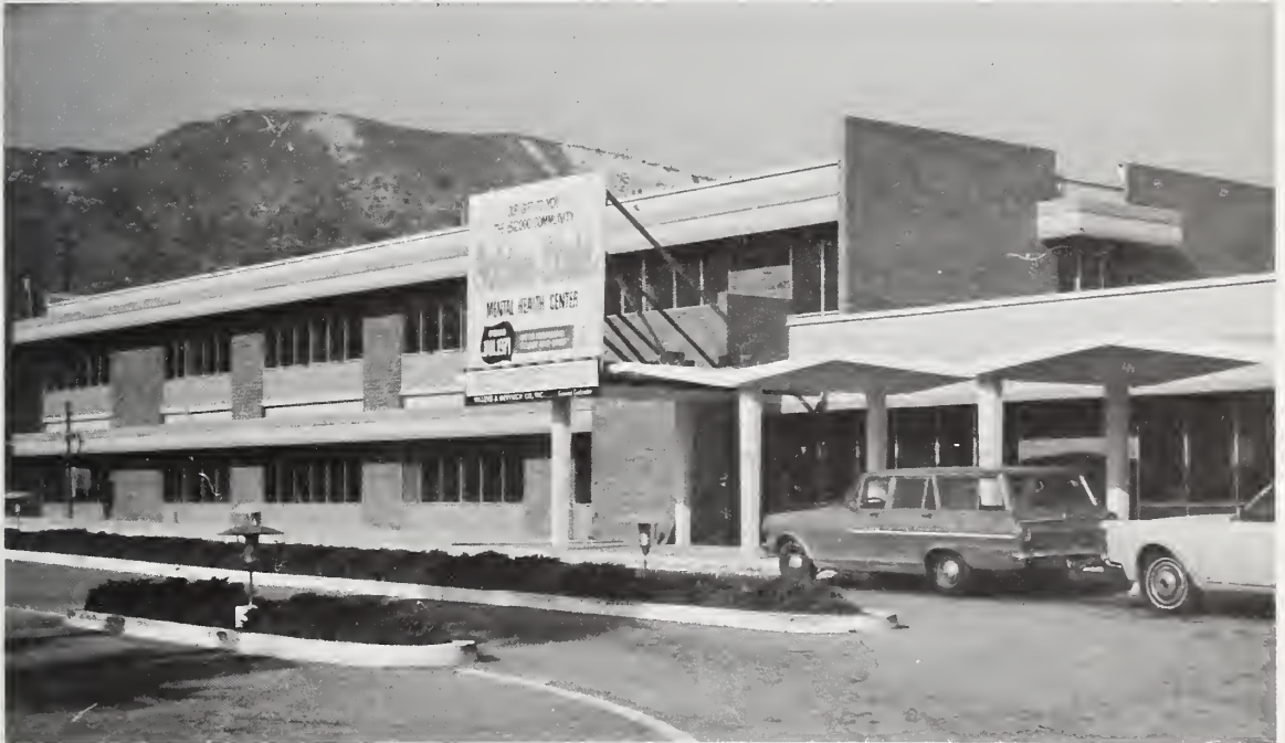
Figure 5.87 New two-story (26-bed) Mental Health Center.
