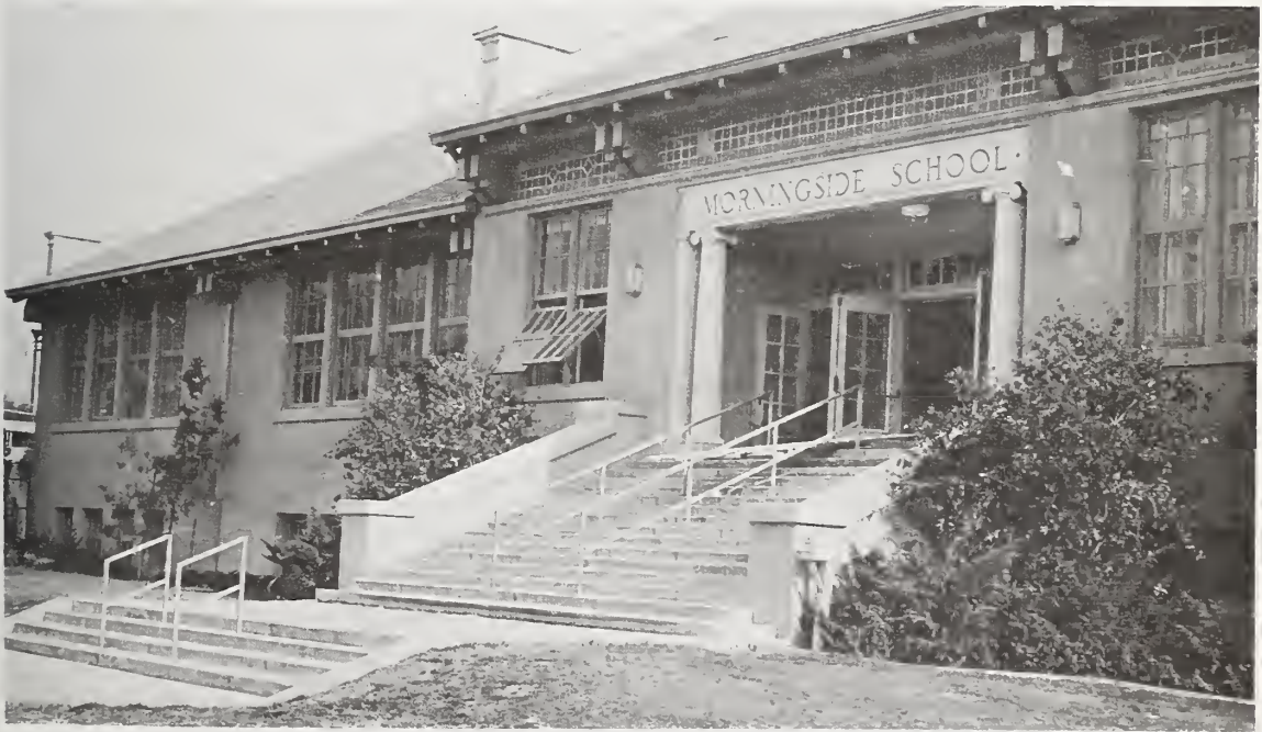
Figure 6.7 Morningside School Building #1 was constructed in 1915 and strengthened to resist earthquake forces in 1964.
