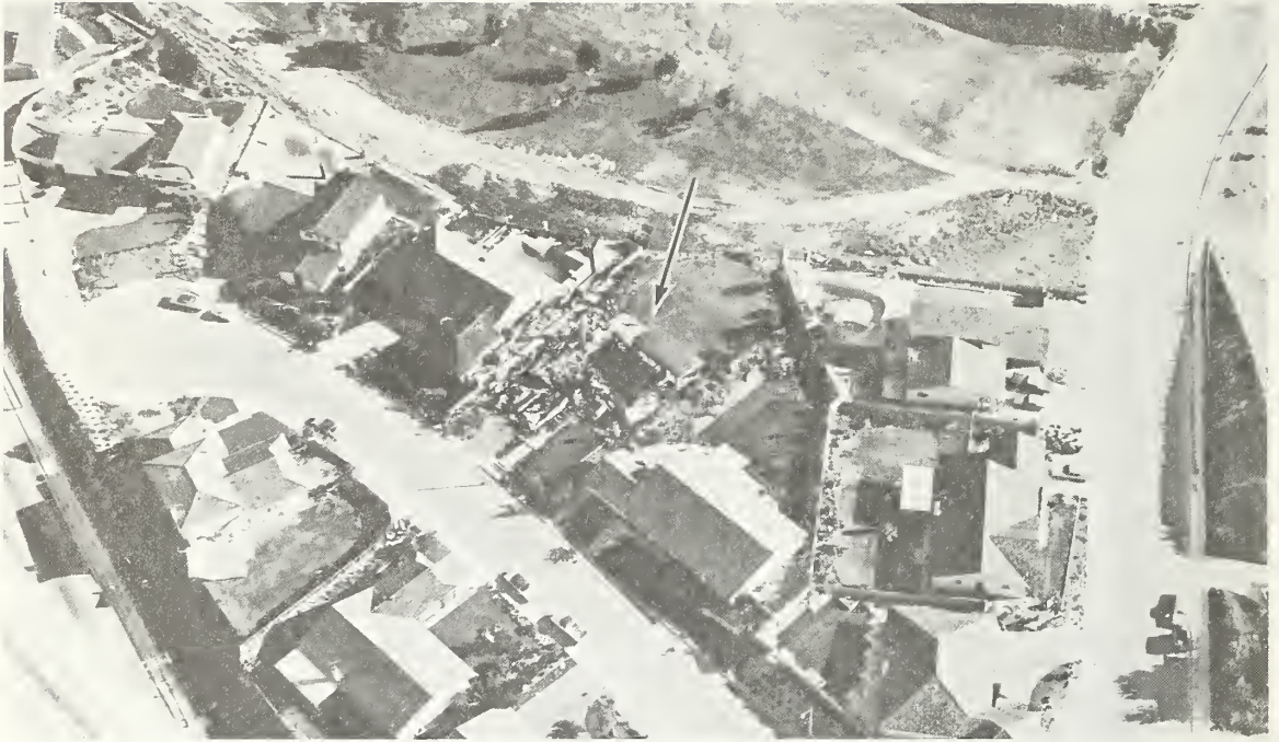
Figure 8.24 House in Knollwood area destroyed by fire.
