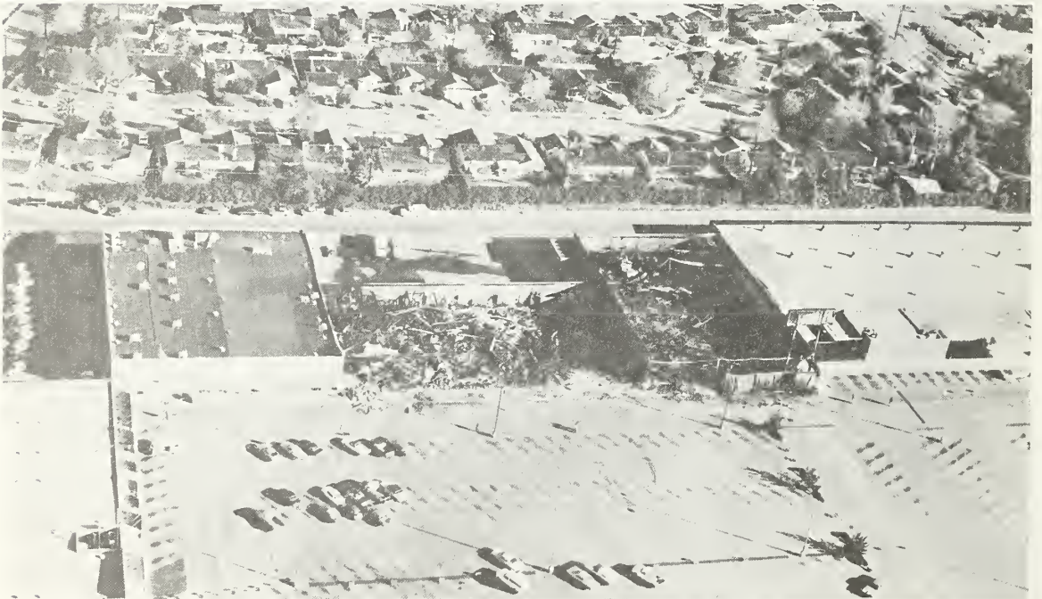
Figure 8.25 Commercial buildings destroyed by fire (Chatsworth Street and Zelzah Avenue, Granda Hills).
