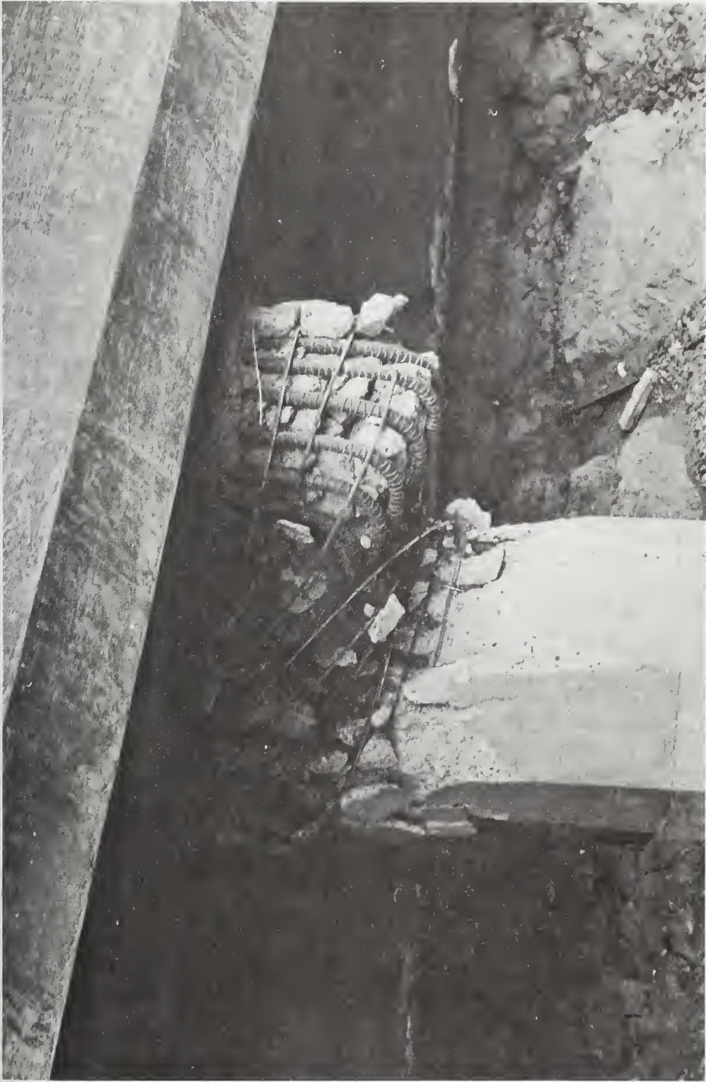
Figure 7.24 Close up of exterior spiral column.
