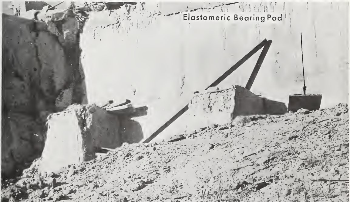
Figure 7.16 Close up of east abutment and elastomeric bearing pad.
