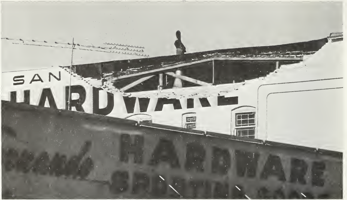
Figure 5.142 Damage to brick masonry parapet wall.
