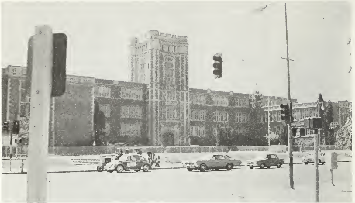
Figure 6.2 Main building at Los Angeles High School before demolition.
