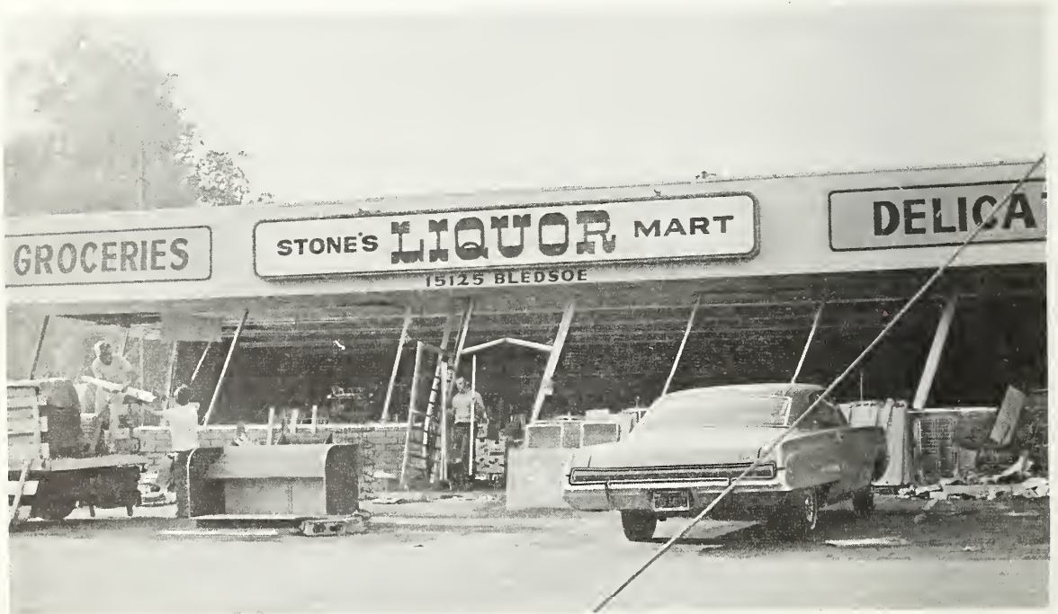
Figure 5.179 This distorted light-frame store is located near the Nethercutt Museum.
