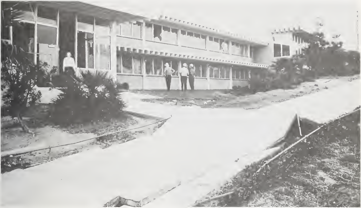
Figure 6.36 Some buildings were constructed with split levels to accommodate a sloping site at the Los Angeles County Juvenile Facility.
