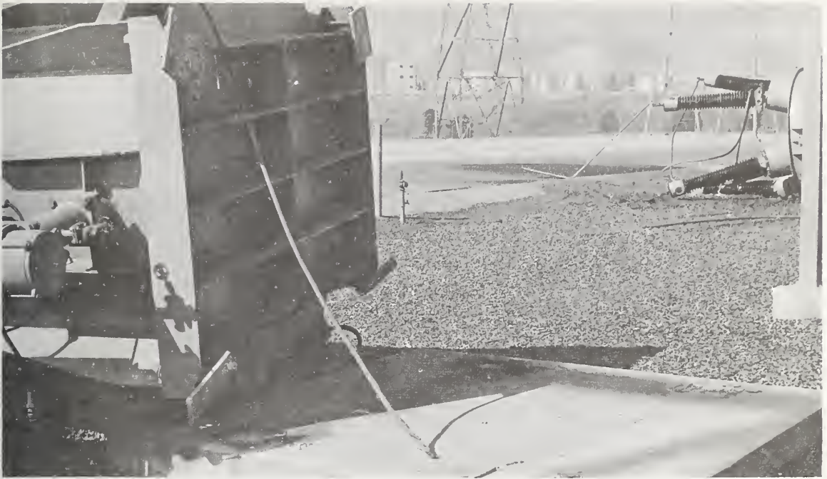
Figure 8.16 View showing bottom of toppled oscillator with its steel base plates and top of the foundation slab.
