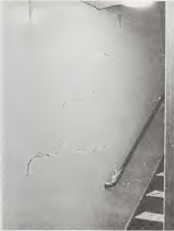
Figure 5.155 Reinforced concrete masonry wall around the Medical Center parking lot. Arrows indicate the location of vertical reinforcement.
