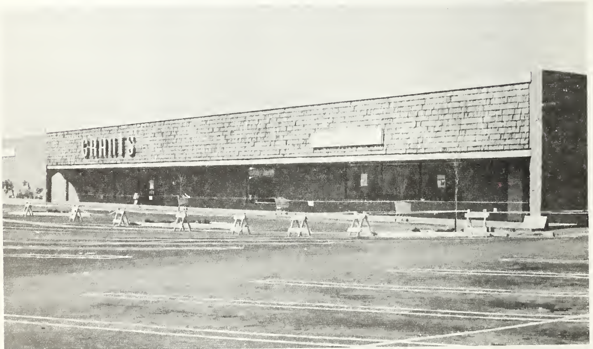
Figure 5.128 Exterior view of Grants Department Store.
