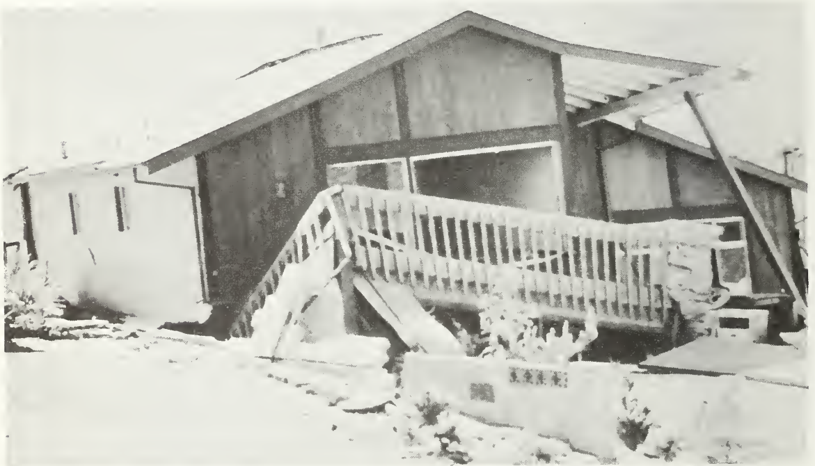
Figure 5.159 Collapsed split-level residence at Almetz Street and Leedy Avenue.
