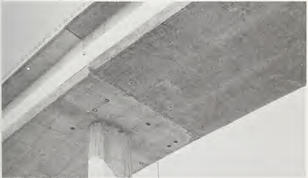
Figure 7.31 Typical movement at a hinge joint of a slender box girder bridge.
