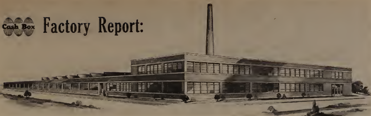
Shown at left—main Bally plant on Belmont Ave., Chicago, Illinois.
