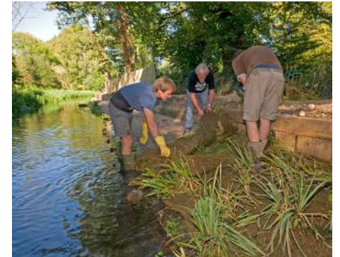
Plants sourced from the Itchen and grown on in a nursery are installed by contractors, providing 'instant habitat'.
