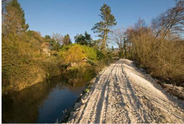
Rebuilding Allbrook's crumbling banks. Image Dennis Bright
