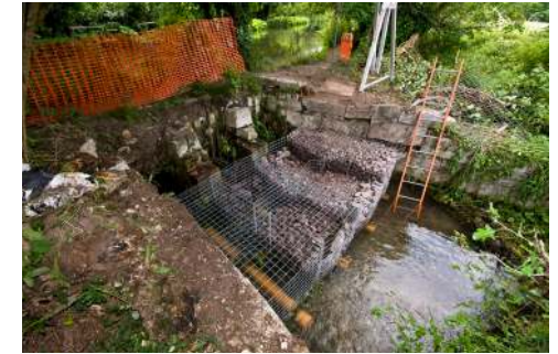
Stone-filled gabions prevent the stonework of Brambridge Hatch from collapsing
