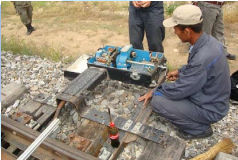
Points inspection and motor maintenance
