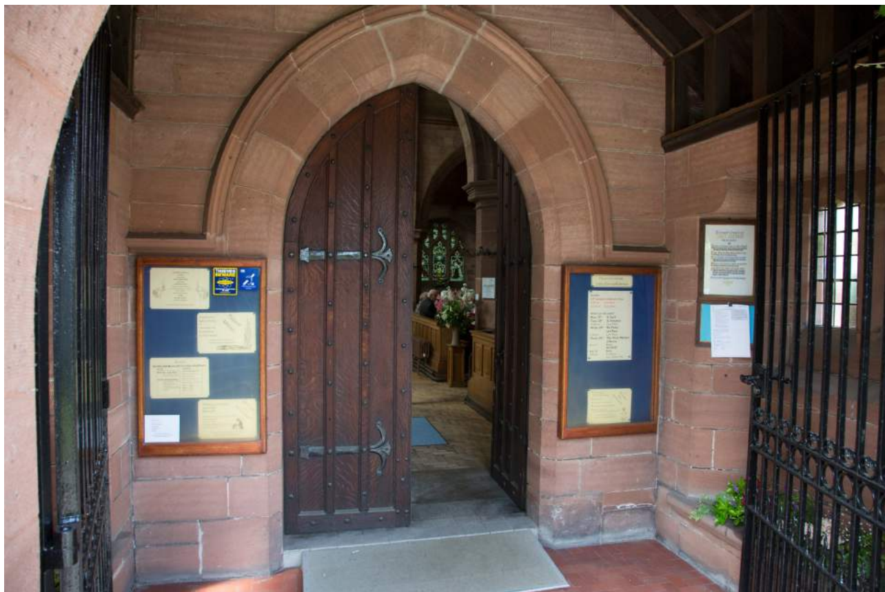
The main entrance porch showing ramped access to the main door
