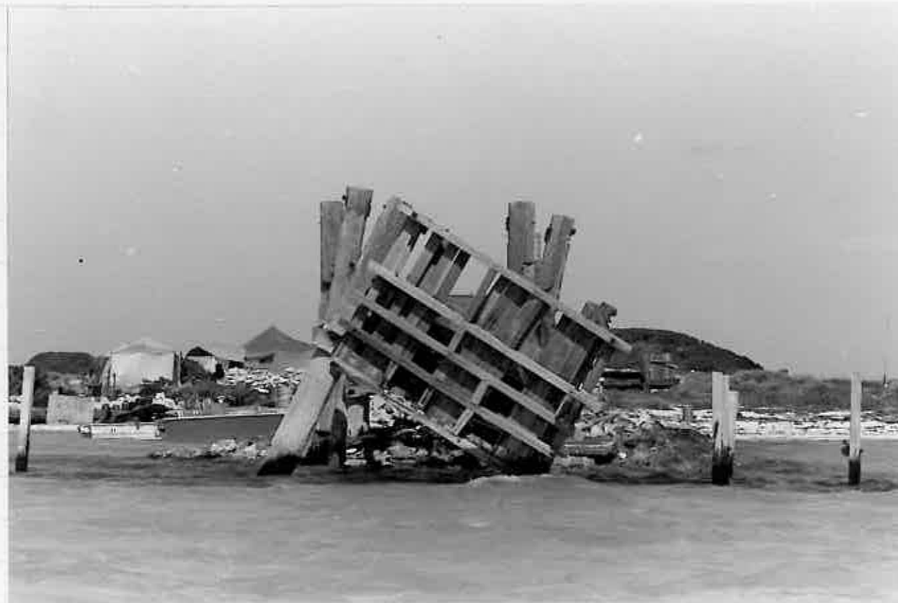
Seaward view of phosphate loading jetty, Pelsaert Island October 1979.
