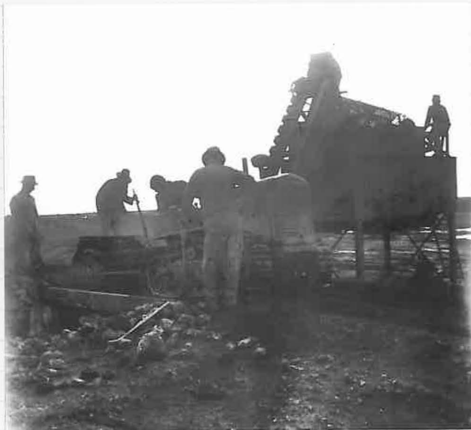
Discharging guano and rock phosphate from scoop into bucket elevator.
