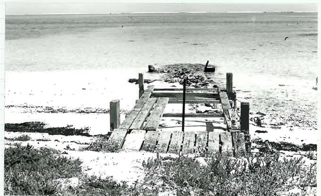
Jetty remains, Pelsaert Island 1979
