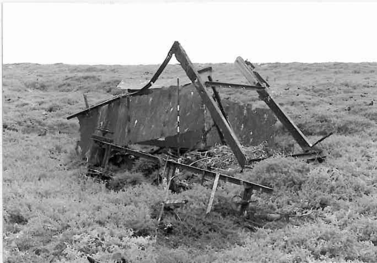
Remains of steel bin on northern guano field, Pelsaert Island, October 1979.
