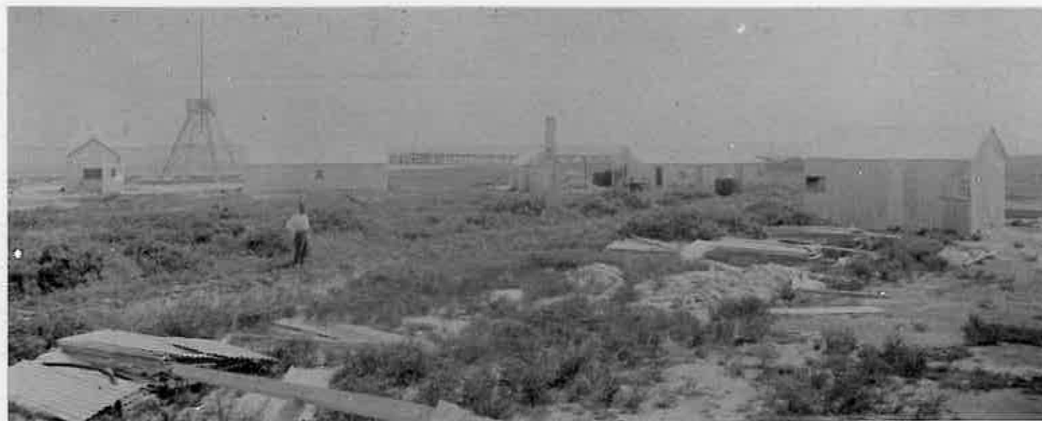
Pilsant Island station and jetty.
