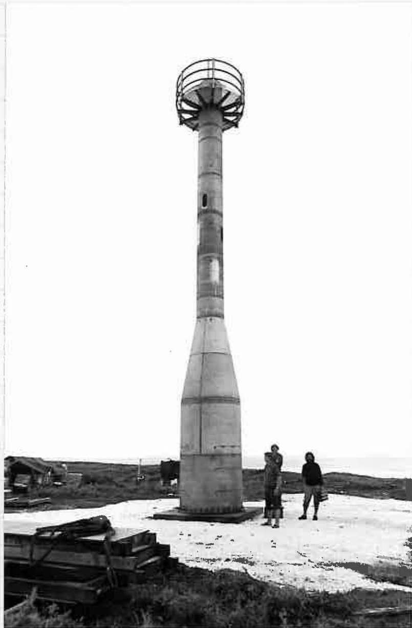
Pelsaert Island lighthouse during the final phase of construction, 1974.
