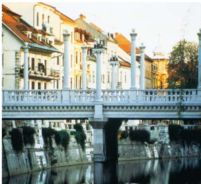
Čevljarški most / Cobbler’s Bridge
