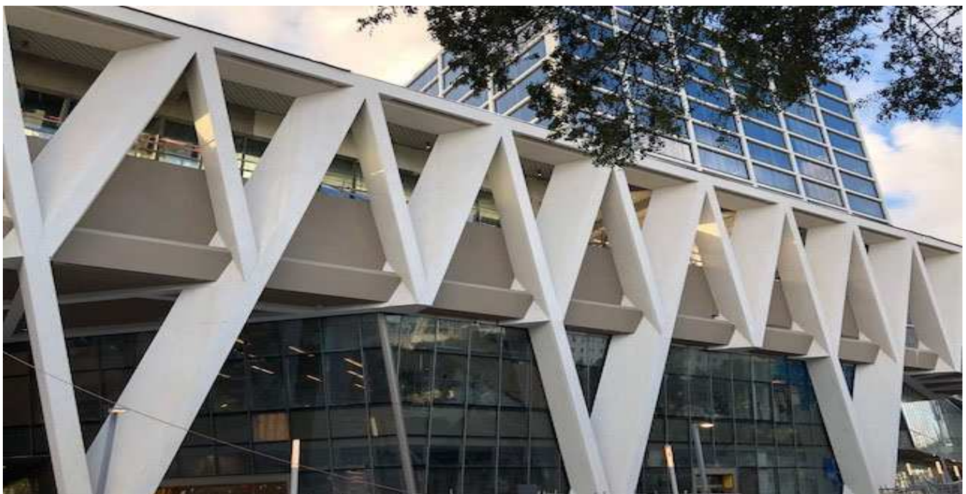
Miami Station Lobby Entrance
