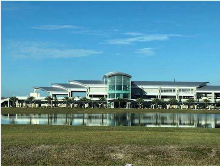
The Intermodal Transfer Facility Exterior
