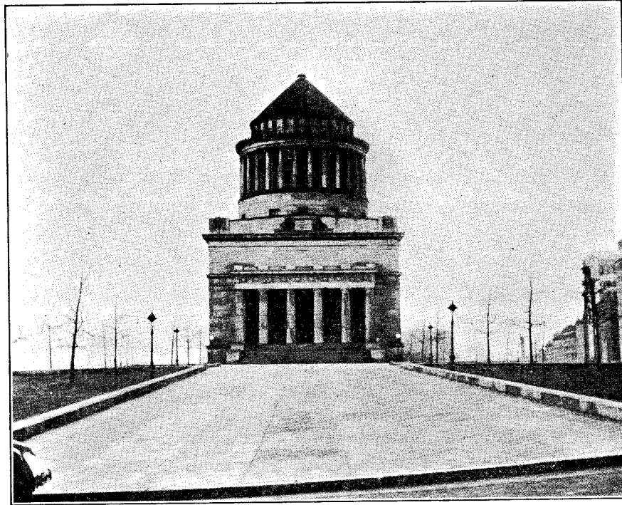
RIVERSIDE PARK New Pavement of Grant's Tomb
