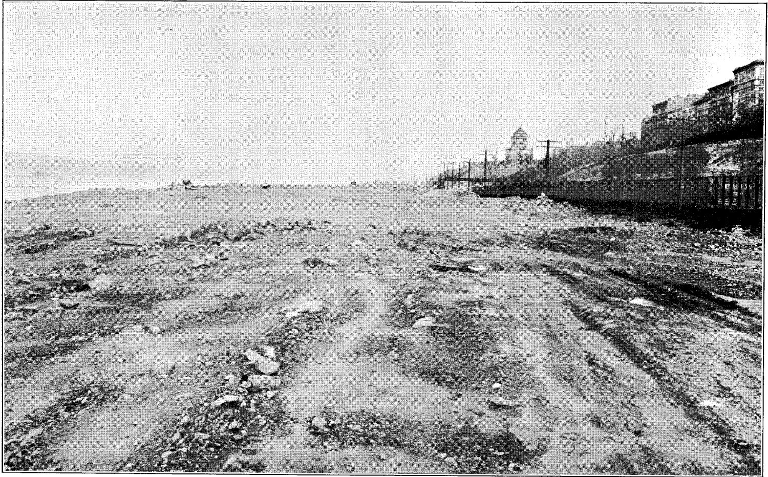
RIVERSIDE PARK, SHOWING EXTENT OF FILLING OPERATIONS Looking North from 110th Street
