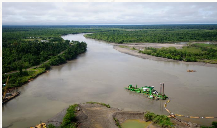
DURING 2008, ALMOST 4 MILLION CUBIC METRES OF RIVERINE SEDIMENT WERE DREDGED AT BIGE BY THE 'CAP MARTIN'
