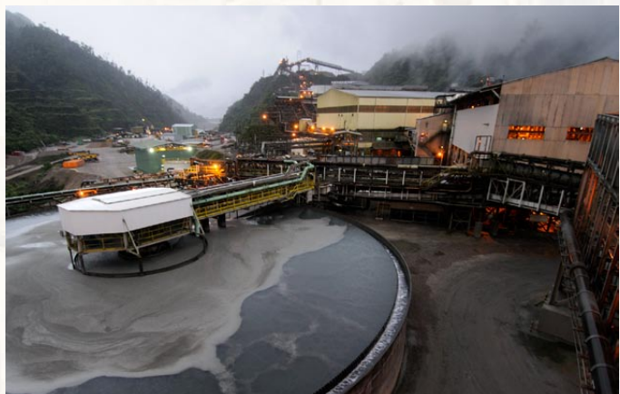
THE TAILINGS PROCESSING PLANT THAT IS PRODUCING A FINAL TAILING STREAM OF 1% SULPHUR AND SULPHIDE CONCENTRATE CONTAINING BETWEEN 42% AND 45% SULPHUR
