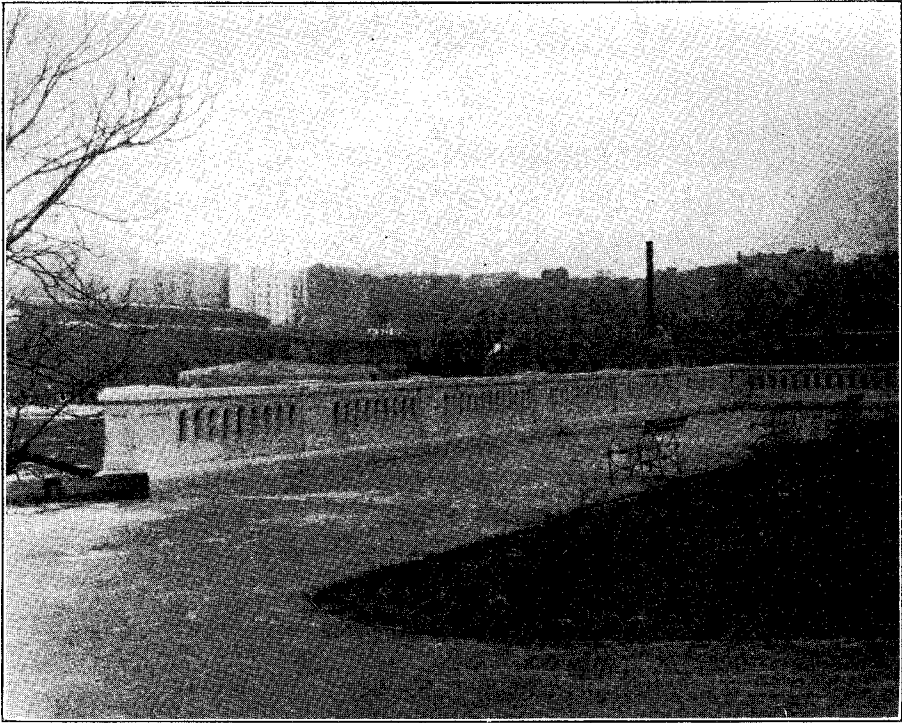
SPEEDWAY—NORTH END NEW CONCRETE BALUSTRADE Harlem River Driveway
