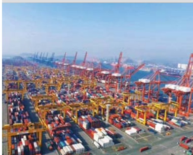
PSA HYUNDAI PUSAN NEW-PORT TERMINAL
