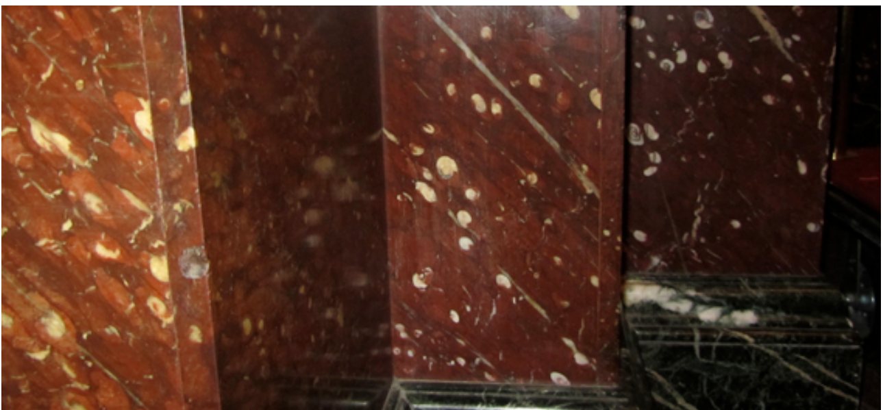
Griotte de Sost, rich in goniatites clads the lower walls above skirtings of Vert des Alpes (just seen at the bottom left).
