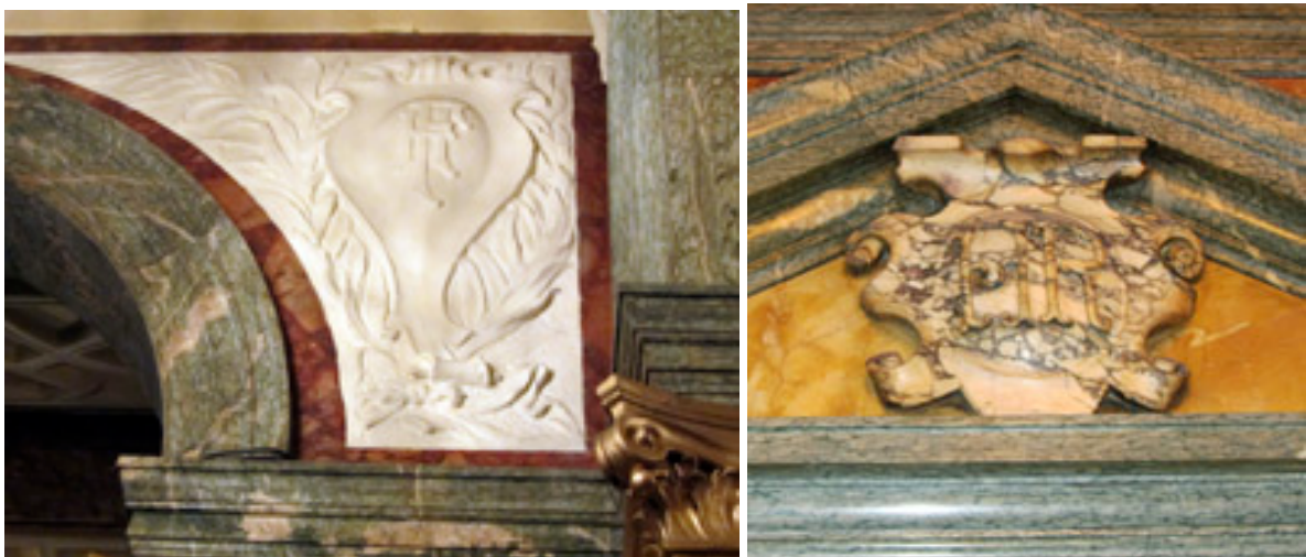
Left: panels of decorative plaster-work are surrounded by borders of Brèche Sanguine; Right: A scrolled medallion with the monogram HR is made of Breccia Violetta on a ground of Giallo di Siena, framed by a pediment of Campan Vert.
