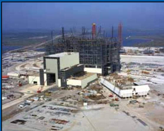
The steel framework of the Vehicle Assembly Building rises on Merritt Island, Fla., during construction of America's Spaceport in November 1964. The low structure at right is the Launch Control Center.
