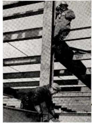
WEWS cameraman sits high to shoot film of Cleveland steel construction worker for part of series, Men at Work, typical of station's locally-originated shows.
