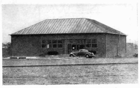
The completed station building. Note the complete absence of any overhead conductors leaving or entering the station. Buried power lines, telephone cable, and an underground r-f transmission line to the antenna make this neat-looking installation possible
