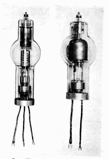
Types of Thyratron and Phanotron tubes used
