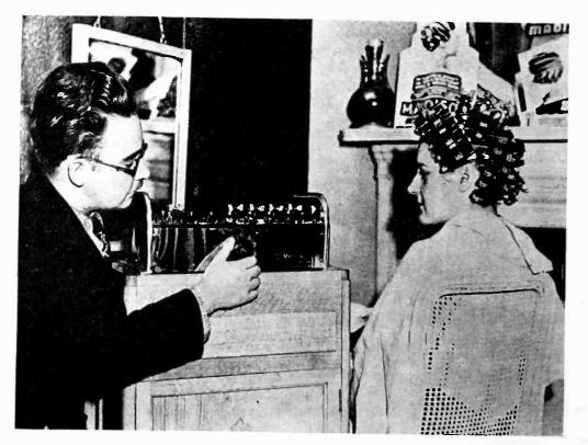
With the aid of electrically-conducting curlers, and in the presence of a highfrequency field, this "permanent-wave" machine in a London beauty-shop avoids heavy wires to operate the heaters
