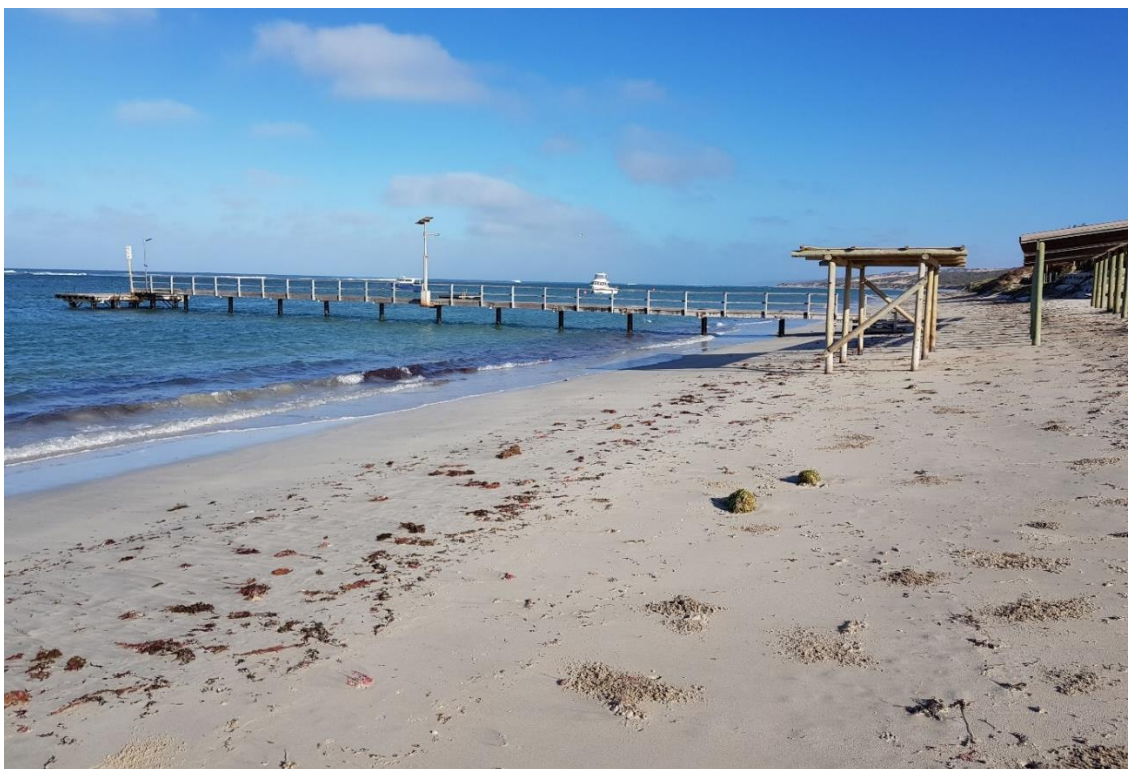
Figure 3-24 Sand beach and jetty. Southern end of Zone 6 looking north.
