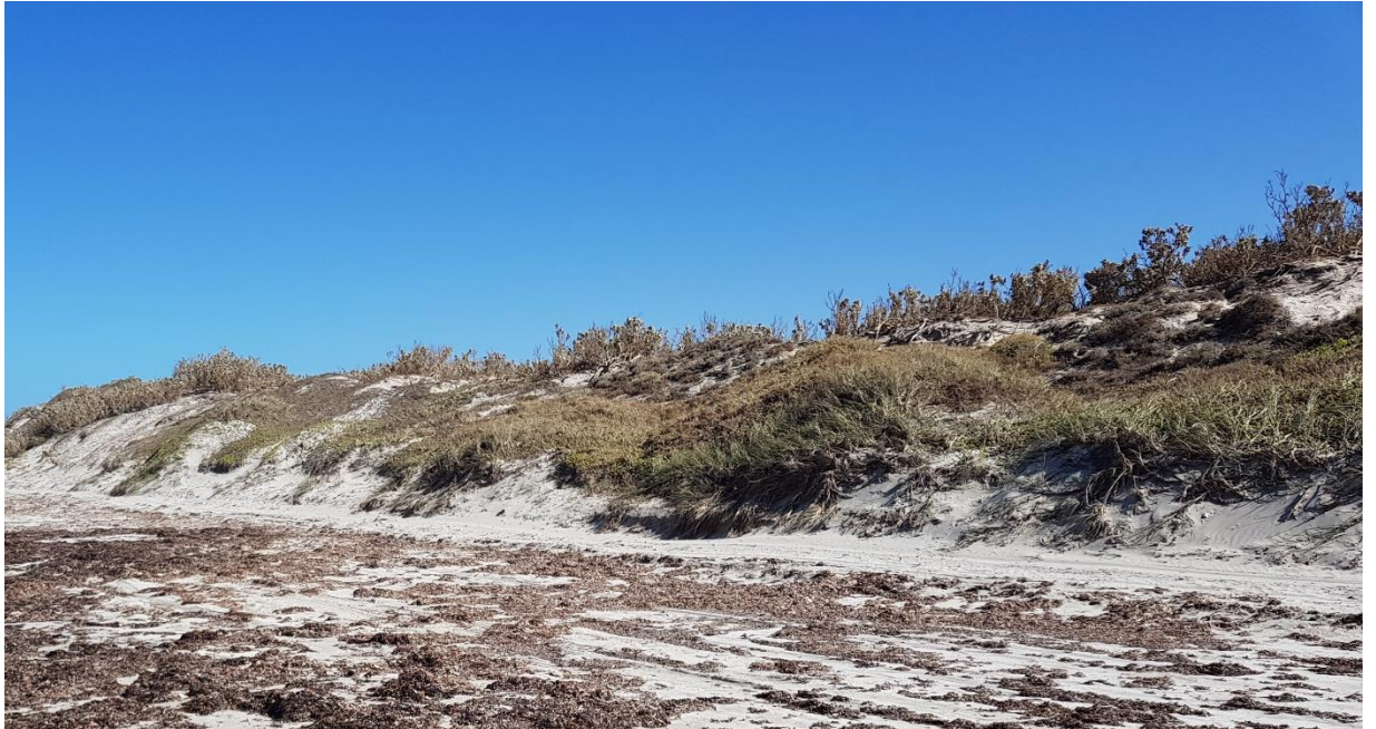
Figure 3-4 Undercut vegetation at base of dune in Zone 2.
