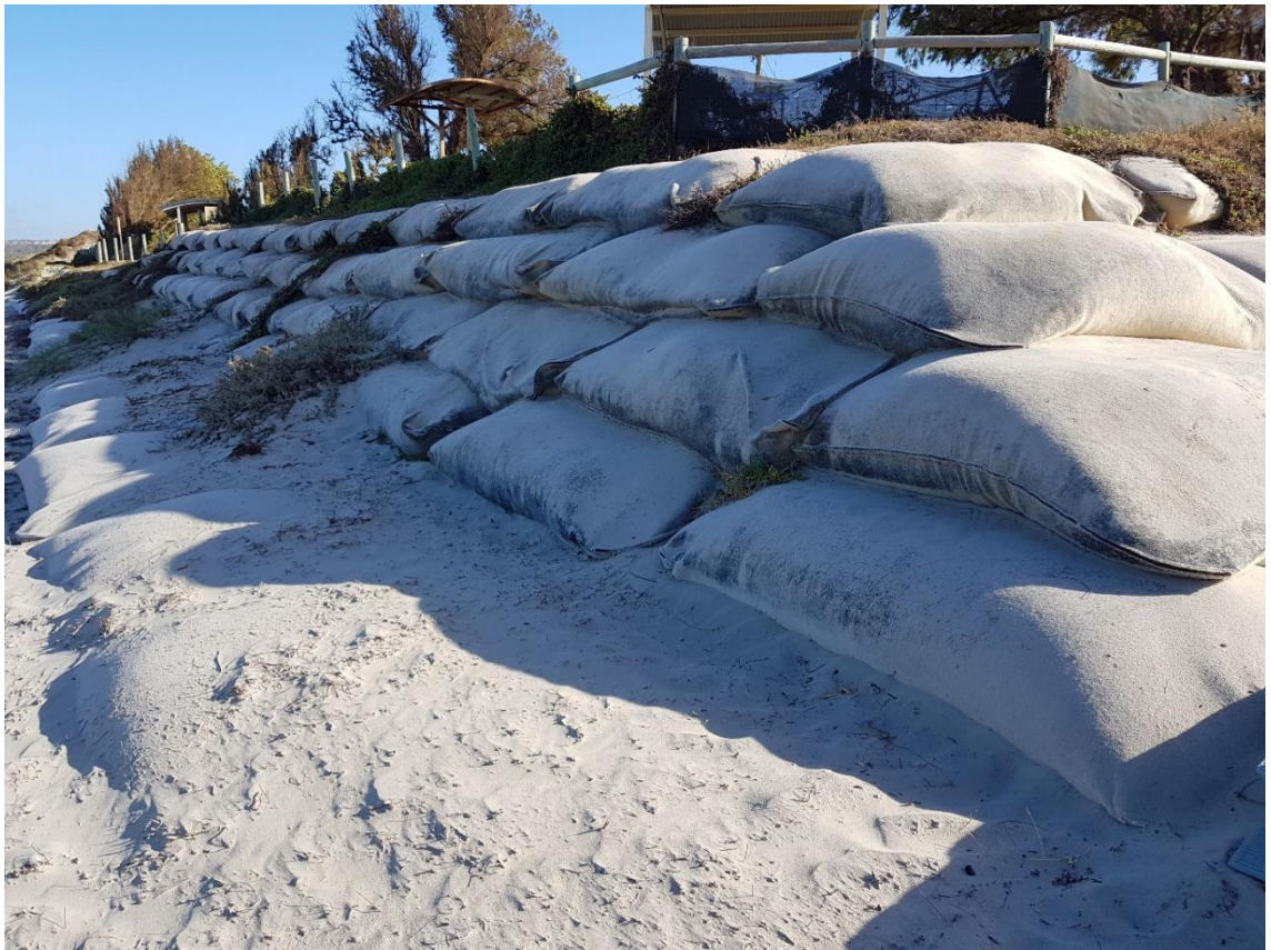
Figure 6 Geotextile sandbag sea wall protection at Horrocks Beach (GHD, 2019)
