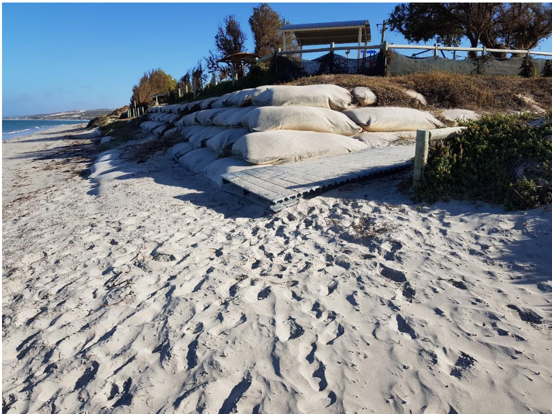
Figure 3-22 Southern extent of GSC Seawall and adjacent beach accesses path.
