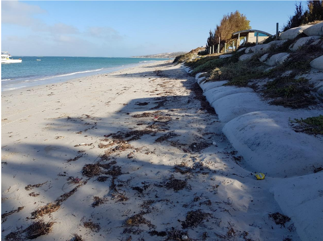
Figure 3-21 GSC Seawall, toe bags still buried by sand, and vegetation and sand covering upper layers.
