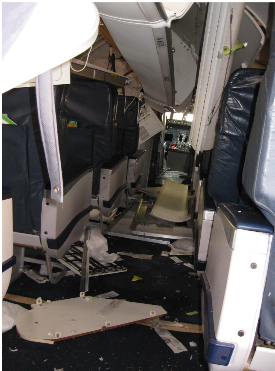
Figure15: Cabin forward of the fuselage break; left stow bins resting over the aisle (looking forward).
