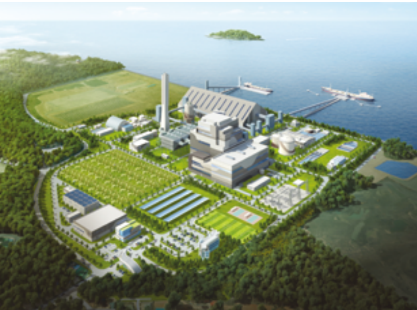
Aerial view of Shin-Seochon Thermal Power Plant
