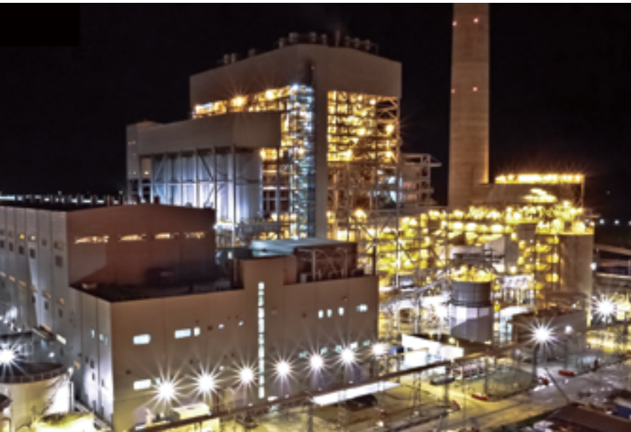
Gheco One Thermal Power Plant in Thailand
