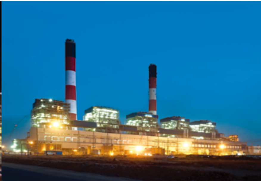
Mundra Thermal Power Plant in India
