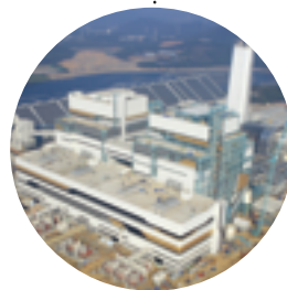
Sinboryeong Electric Generation
