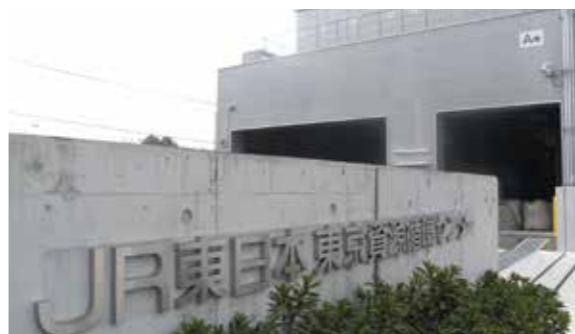
JR East Tokyo Materials Recycling Center
