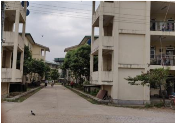
East: Steel Plant Housing Complex
