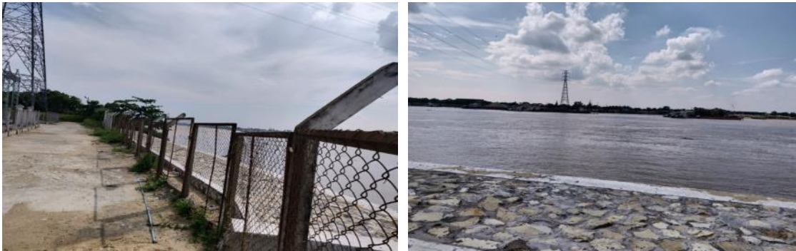
Figure 7.3: Embankment at Ywama Power Plant
