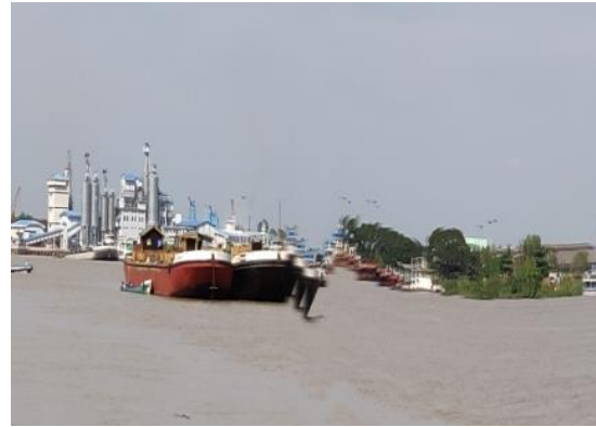
West: Shwe Lin Industrial Zone
