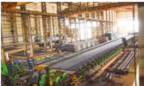
"TMX rebar production line".
