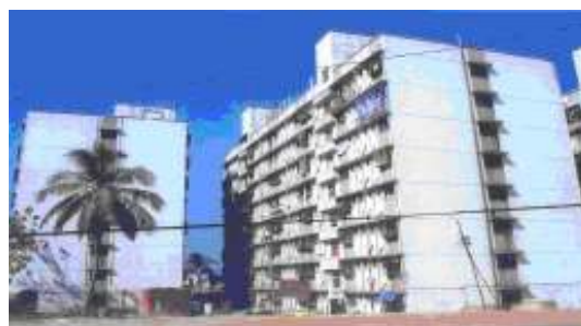
Figure 11: Slum Rehab Housing (MUTP)
