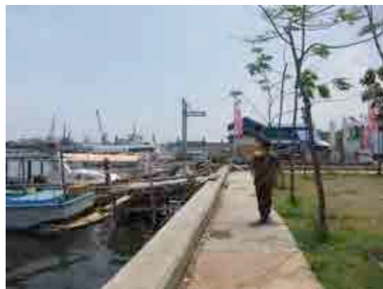
Photo 2: From the west side of the sea tide dike after reconstruction
