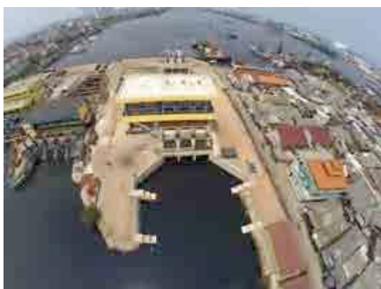
Photo 1: Overall view of the East Pump Station after reconstruction 8
