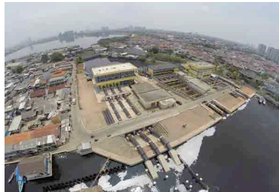
East Pump Station of Pluit after reconstruction 2
