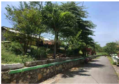
Photo 3: Constructed Levee (Tuban District)
